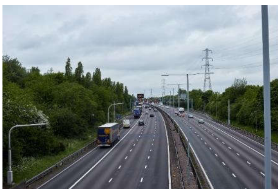
Figure 5-7 Hard Shoulder Running (HSR) in operation
