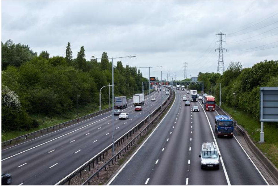
Figure 1-4 HSR with VMSL gantry
