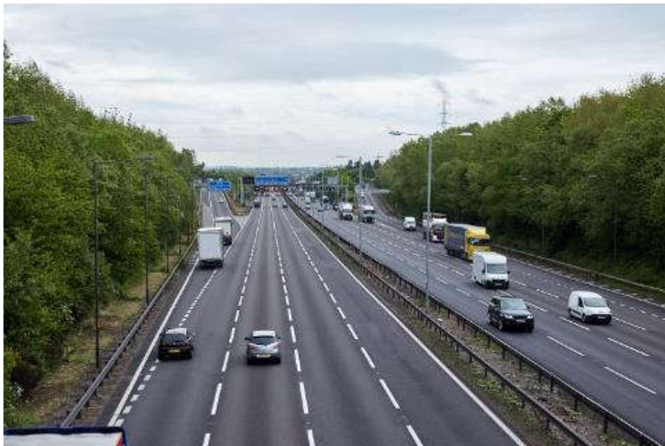
Figure 1-3 TJR (Junction 10) with VMSL gantry
