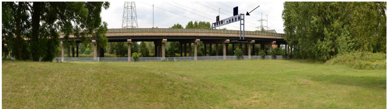
Plate 9.1: Photomontage of the View of a New Gantry from Papyrus Way on the Bromford Viaduct. (178/8+80)
