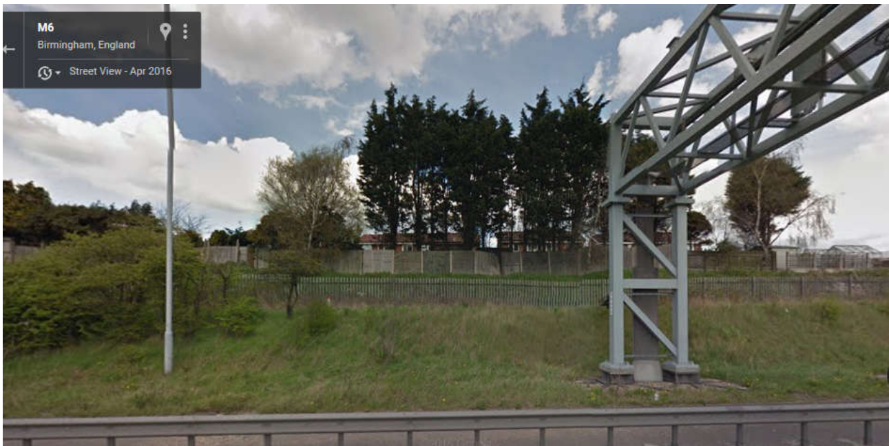
Figure 5-8 View looking towards Grebe Close at gantry 17 – post-construction (April, 2016) Image © Google
