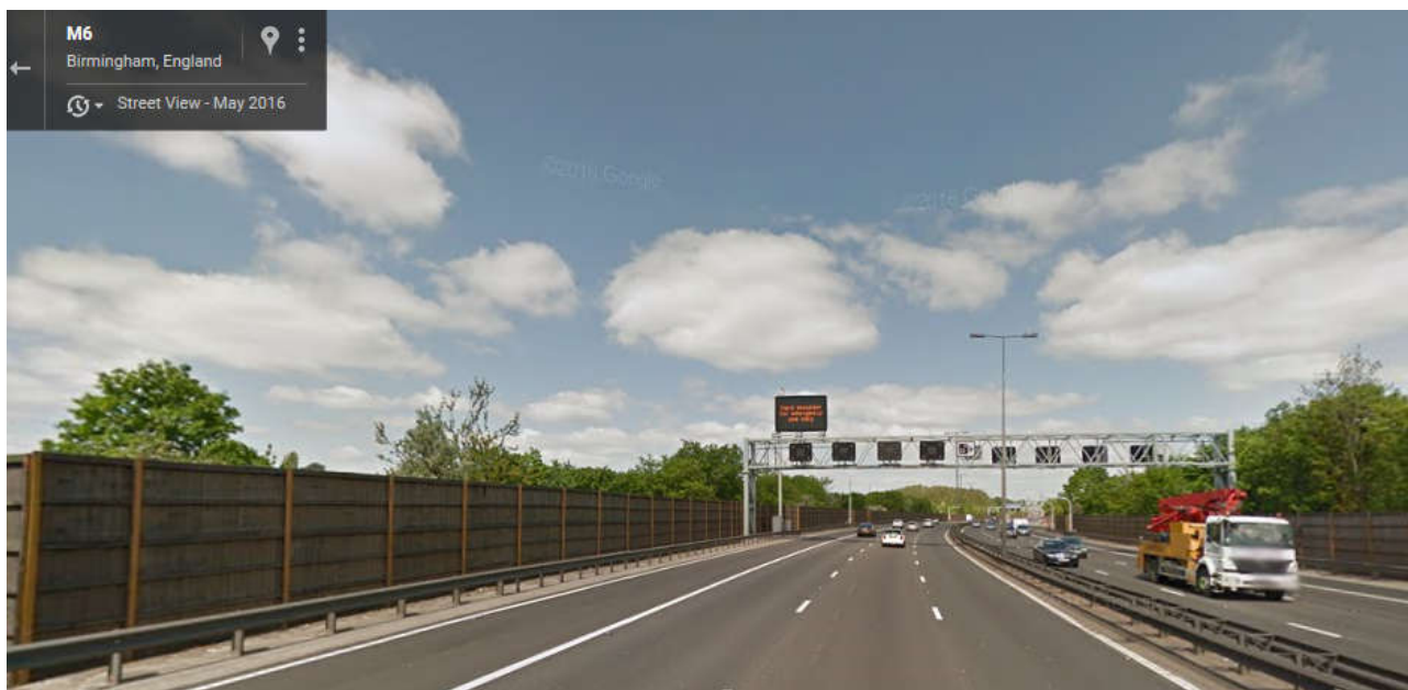
Figure 5-13 View looking northwest at approximate location 188A (J6-7) with noise fence barriers post-construction (May 2016) Image © Google
