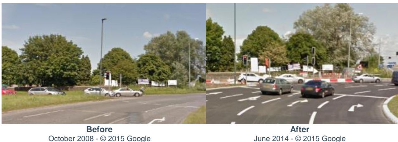
Figure 1-5 M5 Junction 16 Before and After Local Pinch Point Widening Circulatory
