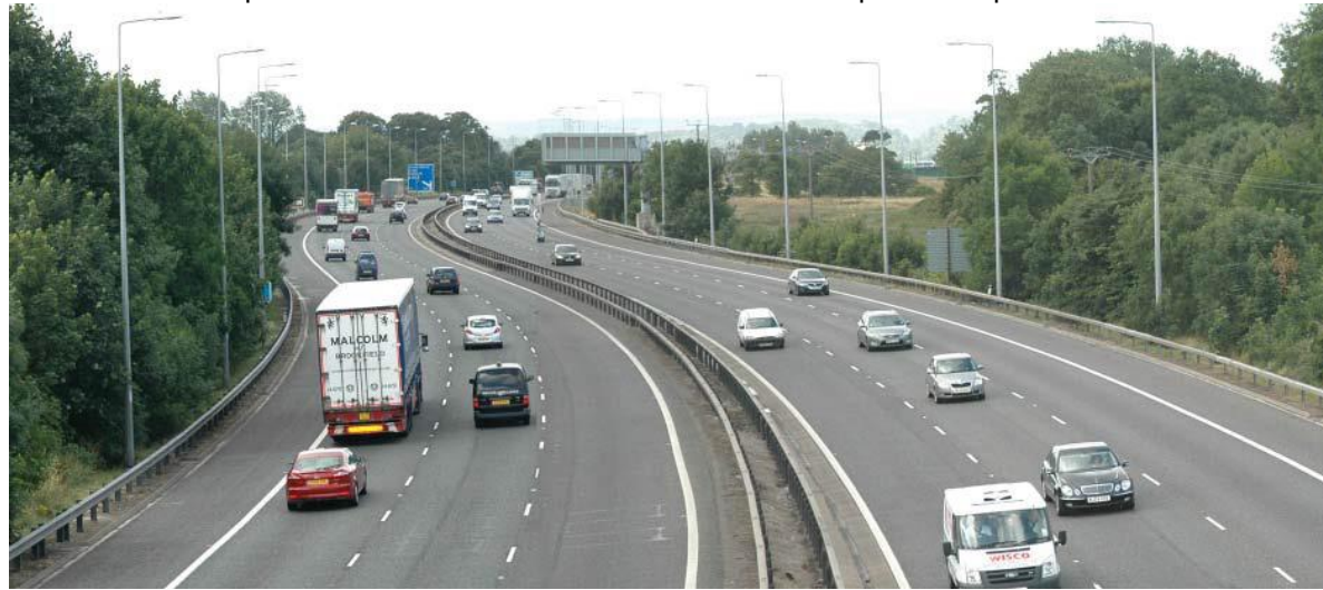
Viewpoint // 17 – before – summer view south from public footpath onto M5
