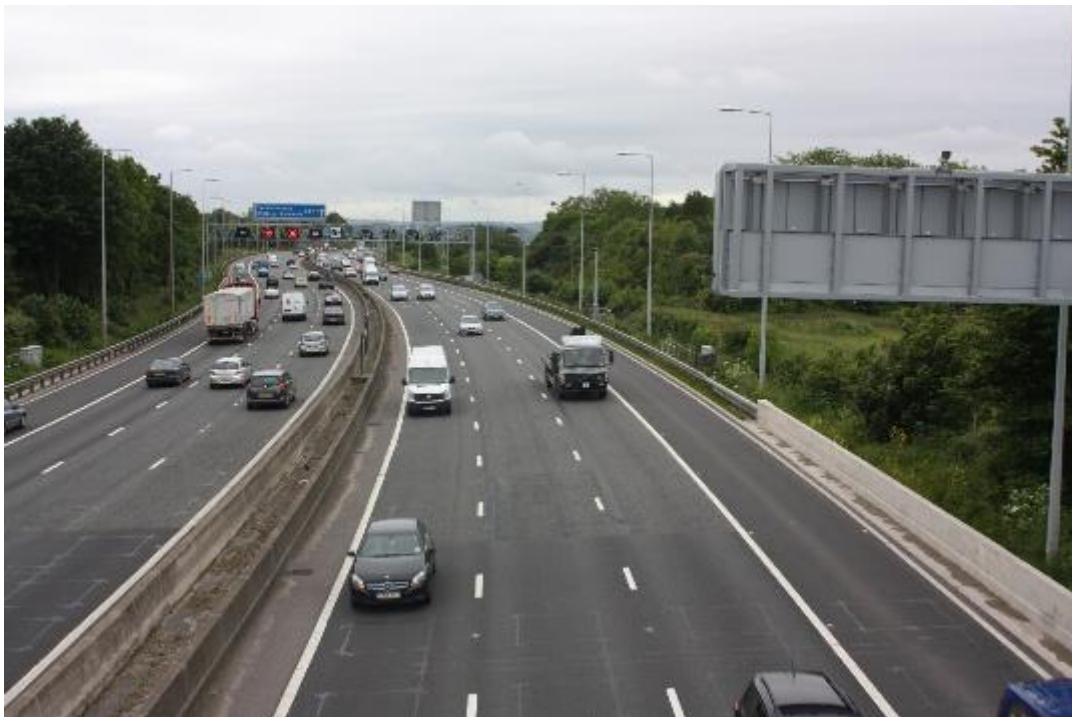
Figure 5-2 New signage and gantries from pedestrian footbridge at Pegwell
