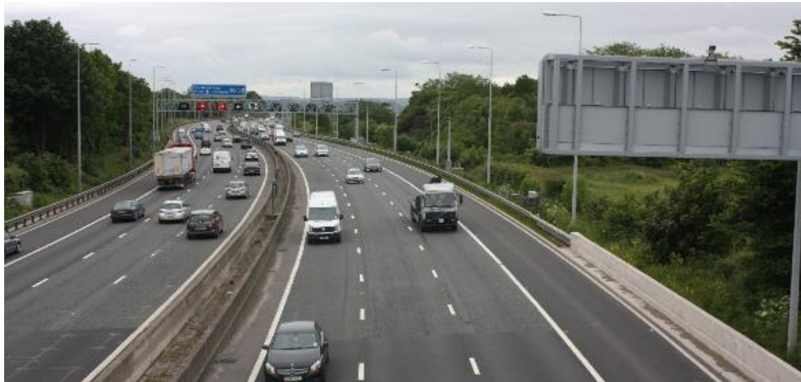
Viewpoint // 17 – OYA – summer view north from public footbridge over M5 towards new gantry superstructure and MS3. EAR stated neutral effect to visual amenity for users of footbridge over M5 near Pegwell Break. View from at footbridge at Pegwell Break is worse than expected at OYA.
