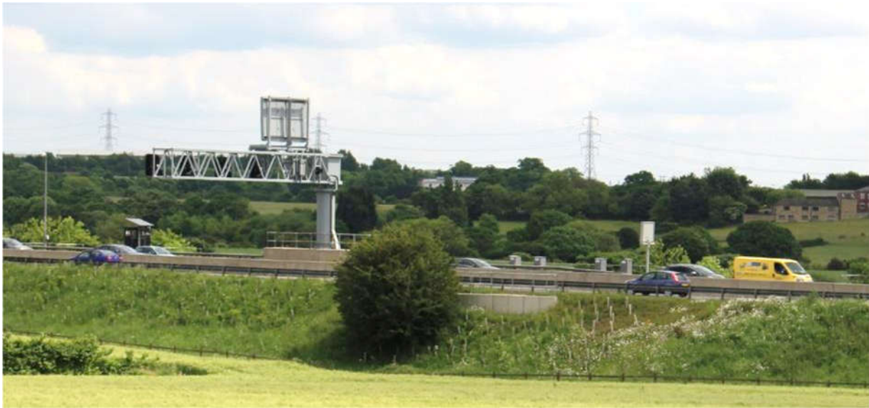
Figure 5-8 Close up of gantry from Woodhouse Lane illustrating mitigation planting in place on embankment slope around a gantry location.
