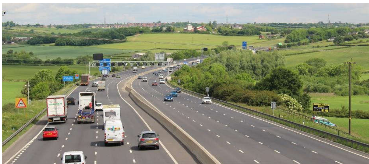
Figure 5-3 View north from Park Mill Lane overbridge with M1 a dominant feature within the rural landscape. East Ardsley on horizon centre, Kirkhamgate to extreme right of view.
