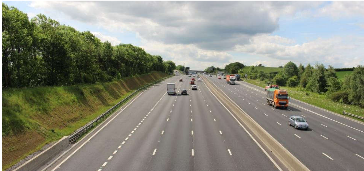
Figure 5-13 Example of soil nailed hydro-seeded slope
