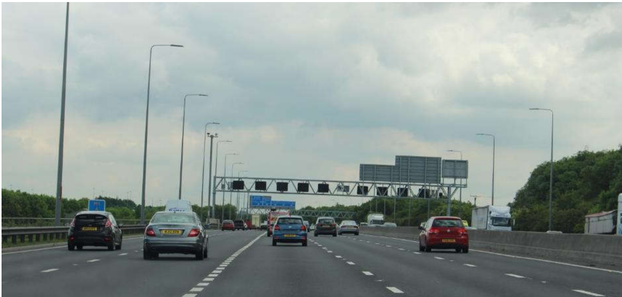
Figure 5-18 Example of new super-span gantry and signs northbound approaching J42
