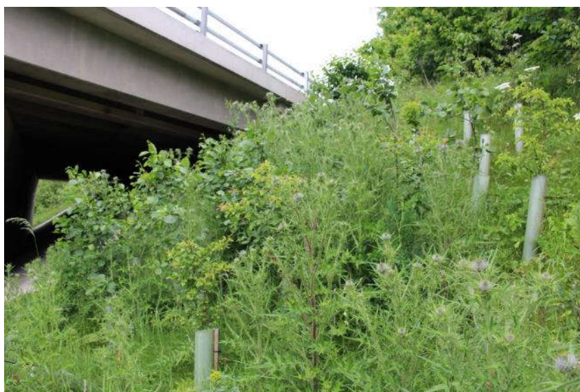
Figure 5-12 Weed growth evident within small planting plot on embankment slope at Lawns Lane with M1 on overbridge
