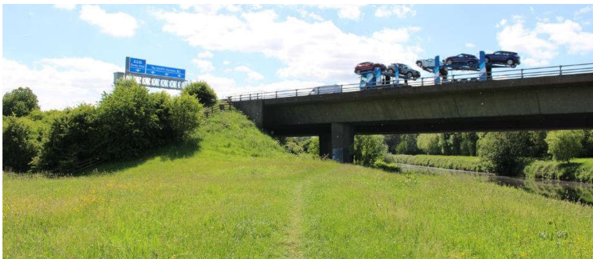
Figure 5-2 View west from public footpath alongside the River Calder; new gantry signs prominent with M1 on embankment and river crossing.
