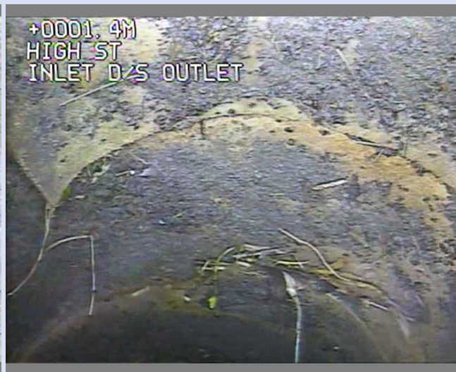
Repair needed in pipe from 11 to 1 o'clock
