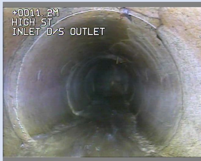
Crack in pipe at joint, from 7 to 1 o'clock
