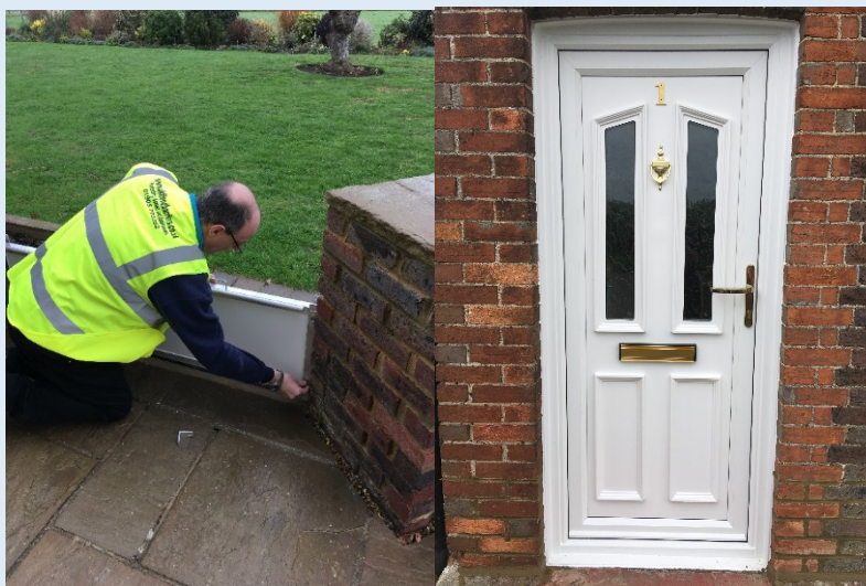
Photos left and right, examples of flood resilience measures: flood gates, flood door and non-return valves
