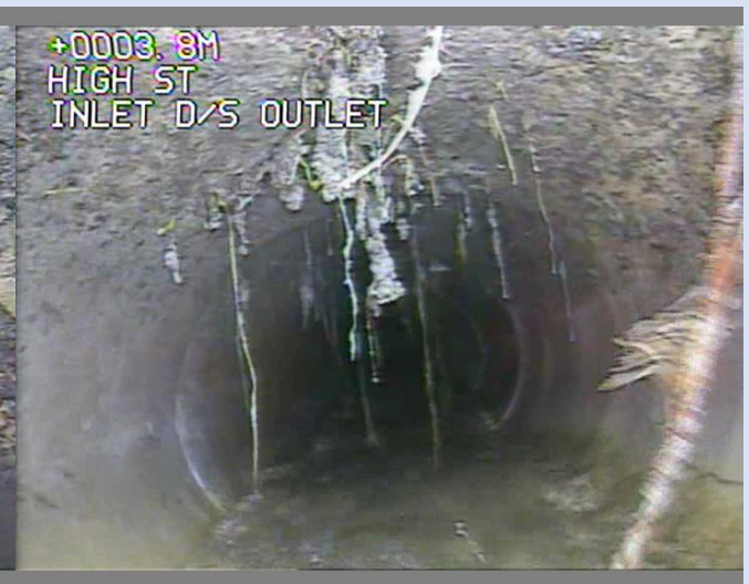
Fracture, longitudinal, at 12 o'clock
