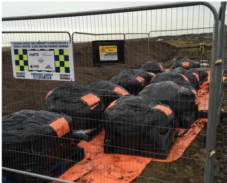
Figure 6 Storage of bagged radioactive contaminated soil in a secure compound
