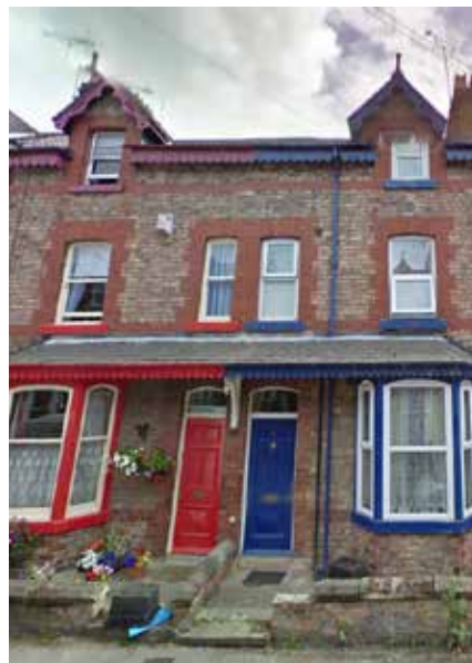
Repeated building features: different colours used for visual interest
