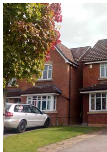
Ample defensible space, incorporating front garden and parking
