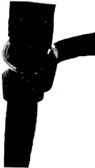
Figure 63: Correct attachment of insulation support strap
