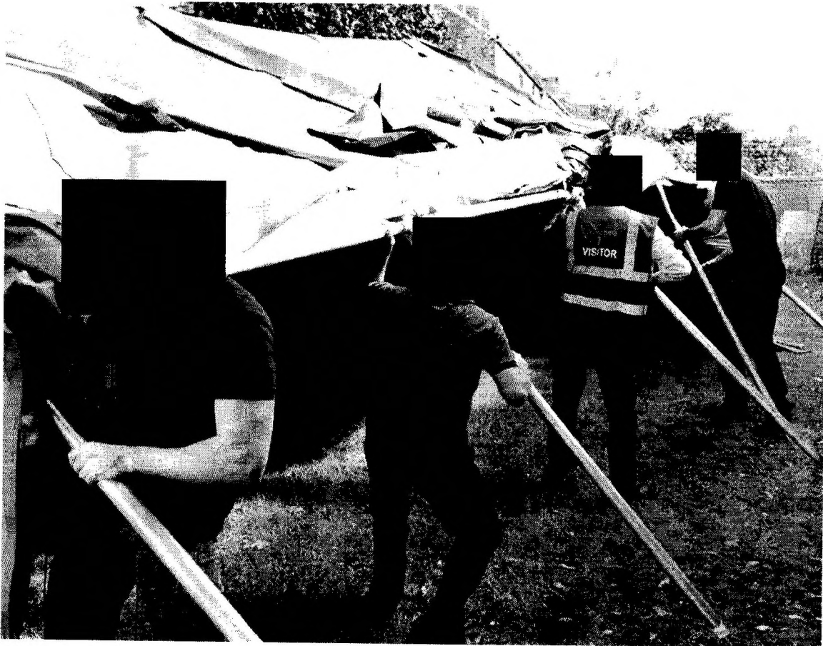
Figure 44: Install the legs on the other side of the tent
