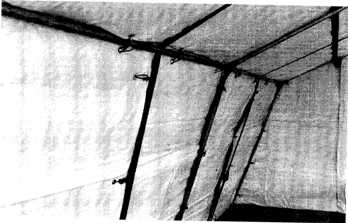
Figure 66: Wall insulation panel (Typical arrangement)
