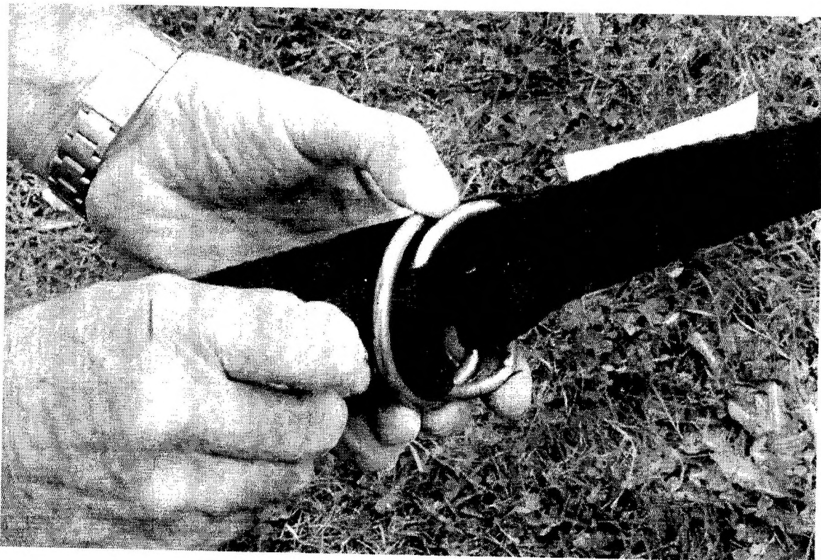
Figure 12: Secure Roof Restraint Strap through rings 2
