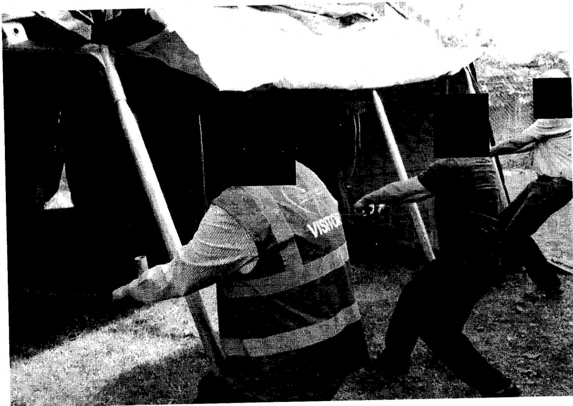
Figure 45: Tug on the base restrain strap to adjust the gap between the legs
