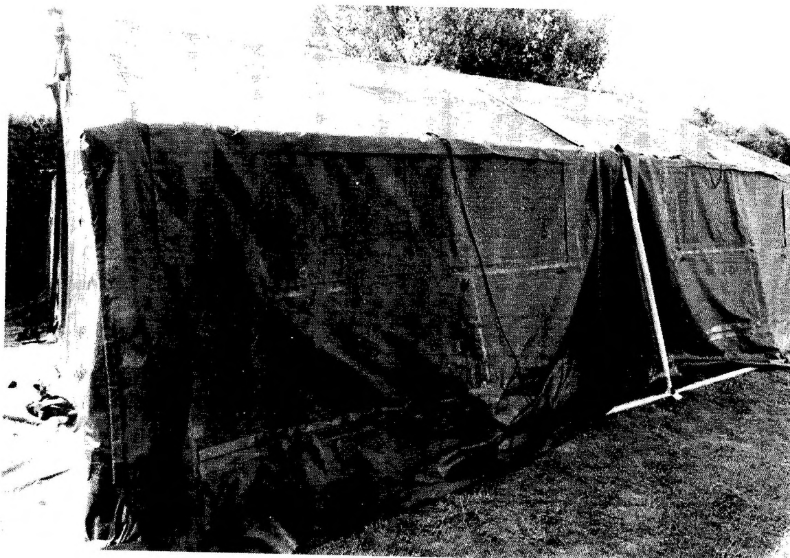
Figure 48: Tent ready for connecting side walls
