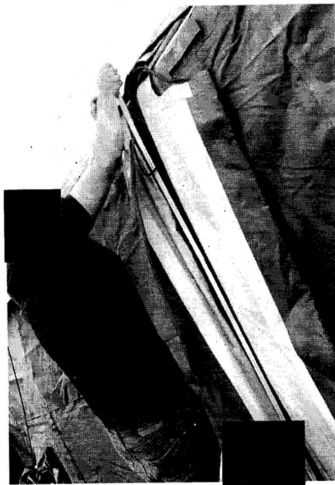
Figure 49: Installing wall keder using two (2) people
