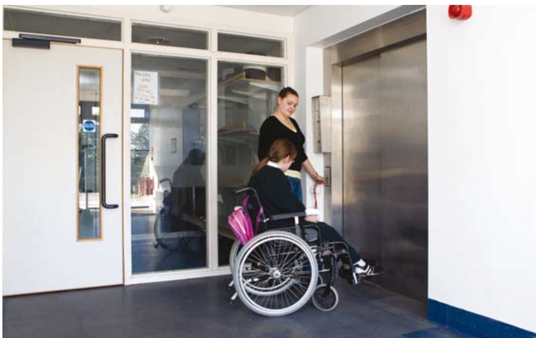
Waiting space outside a lift should take account of nearby door openings and passing traffic.
