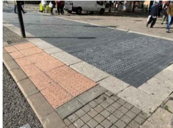
Badly worn blisters at controlled crossing with stem formed from metal studs, many of which are missing
