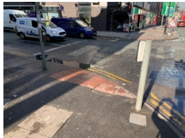
Blisters at signalised crossing with no stem and significant section well below 800mm in depth.
