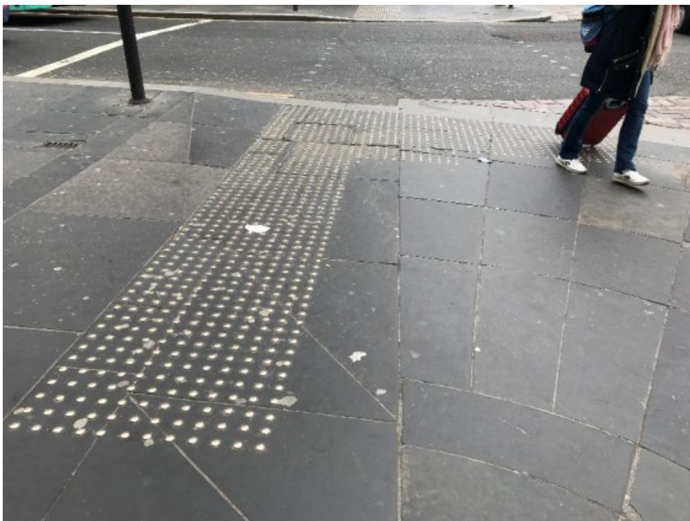
Figure 4: Blister surface formed of metal studs set into stone slabs. One-off public realm scheme in heritage area.
