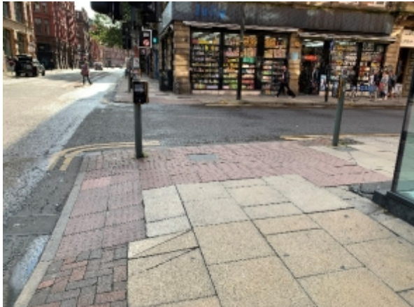
Confusion between stems at closely-associated perpendicular crossings.
