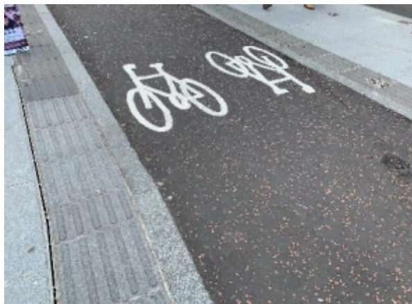
Guidance path surface (400mm depth) used to delineate the edges of a footway level cycle track
