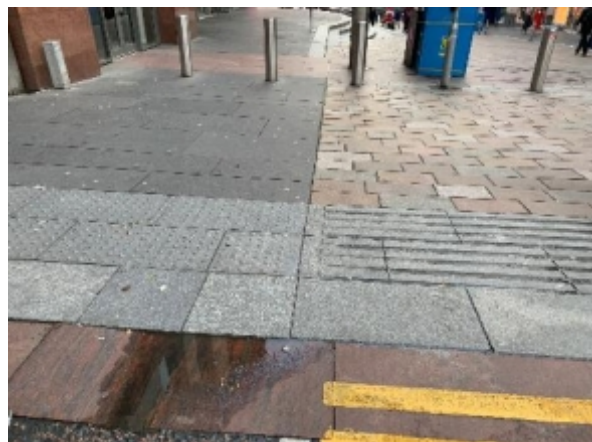
Blister paving at a signalised junction alongside non-standard ribbed paving over nominal vehicle path
