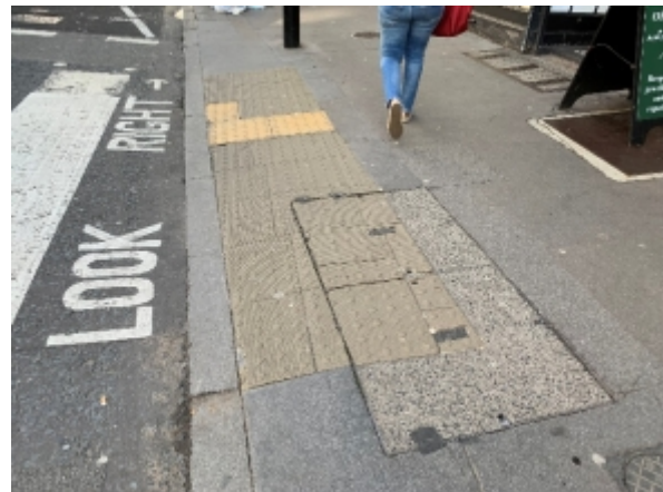
Poorly-contrasting stick-down tactiles at a zebra: helps cover utility trays, but no stem.
