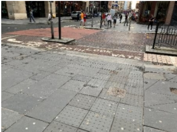
Non-contrasting blisters used for both edge and stem at a signalised crossing
