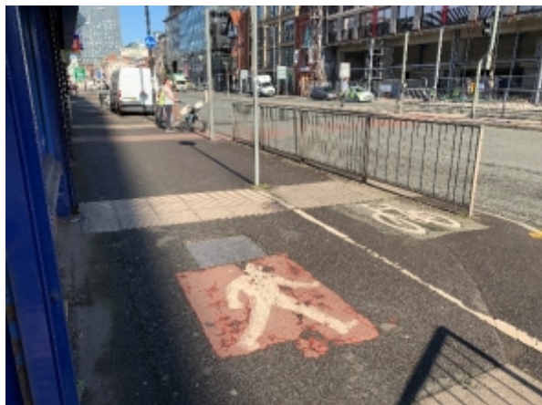
Badly specified parallel footway/cycleway: corduroy used in place of ladder and no delineator strip.
