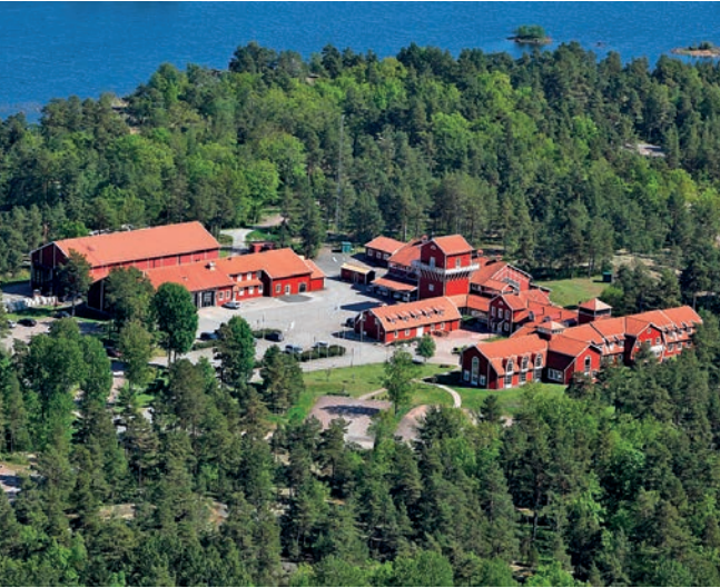
Surface facilities at Aspo Hard Rock Laboratory, Sweden (picture from SKB)
