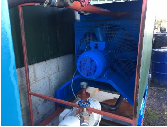
Figure 22 - External radiator, fan & water pump
