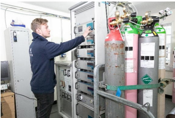
Figure 12 - Signal Gas Emissions Towers
