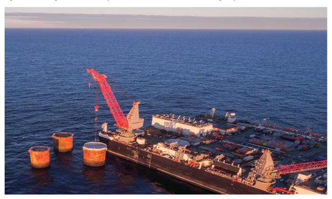
Figure 21. Condition of the Brent Delta GBS after removal of the topside and the fitting of leg caps and AtoN.
