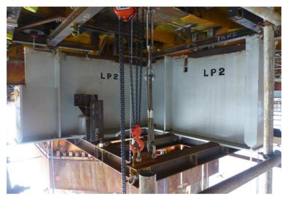
The topside required strengthening with additional steel in order to bear the forces that would be exerted during removal. A significant number of steel doubler plates were welded in place on the primary steel bulkheads of the Module Support Frame (MSF); this required the removal of some local obstructions.
