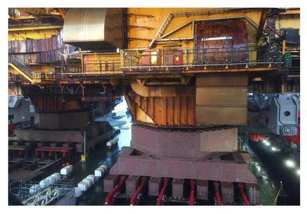
The barge was towed by four tugs to Quay 6 of the ASP facility. Because the barge required a high tide to enter the Seaton Channel and into the dock at Quay 6, it was initially towed to the sheltered 'Turning Circle' in the River Tees, to wait for the appropriate state of tide. At the ASP facility it was moored with its stern to the quay and then carefully ballasted until it rested on the pre-installed grounding pad (Figure 27 and Figure 28). Ballasting was
