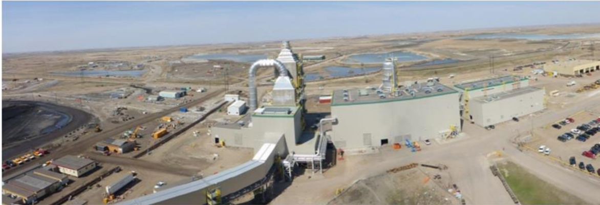
Figure 13-2: SaskPower Boundary Dam Facility (Image courtesy of Cansolv Technologies Inc.)
