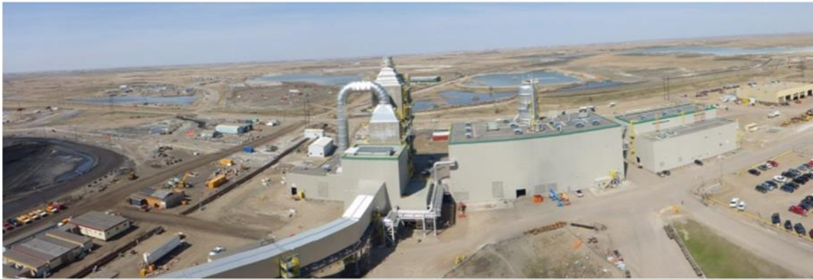
Figure 8-2: SaskPower Boundary Dam Facility (Image courtesy of Cansolv Technologies Inc.)
