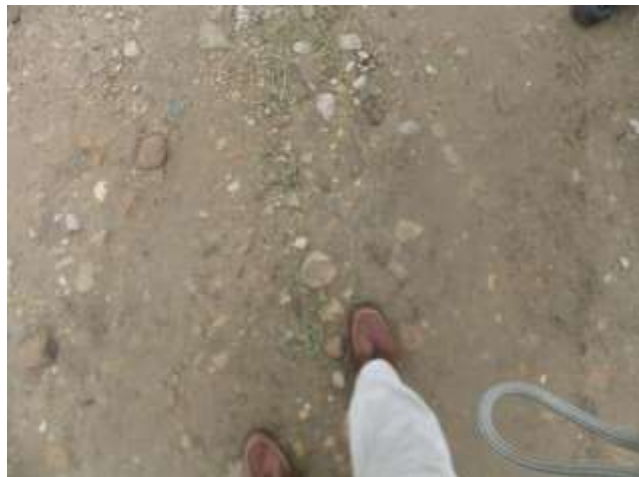
Figure 25 Power house road showing oversize
