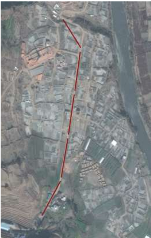
Figure 20 Roughness on Power house road
