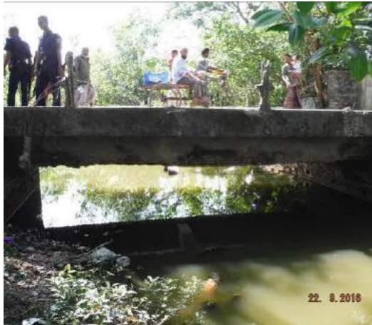
(a) Burridang WFC road bridge
