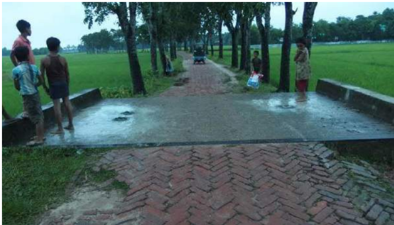
Figure 3-12 Concrete culvert at Boakhali road, Islamabad Union
