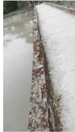
(b) Longitudinal cracking on wheel guard and disappeared rail posts
