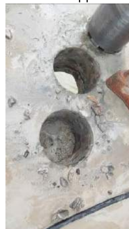
(d) Core hole showing large voiding in the deck slab concrete
