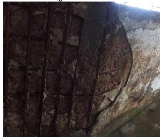
(d) Spalling of concrete and exposed reinforcement underneath staircase
