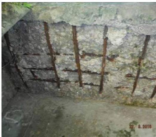
(c) Concrete spalling, exposed reinforcement at deck slab soffit
