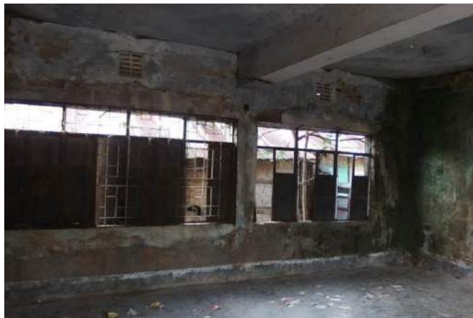
(c) Cracking, delamination and spalling of concrete, mould growth on walls in class room
