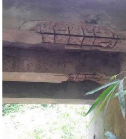
(b) Concrete spalling and corrosion of exposed rebar in girder
