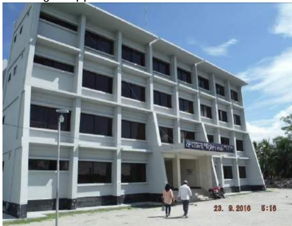
(a) LGED Upazilla Office, Rampal
