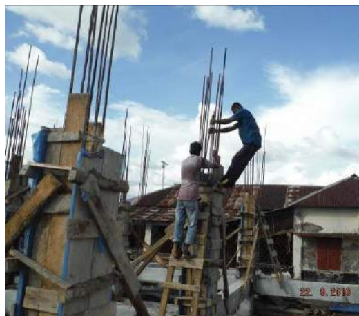
(d) Manual placement and compaction of concrete in a column
