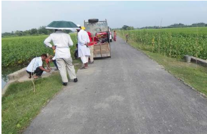
(a) General view of the box-culvert
