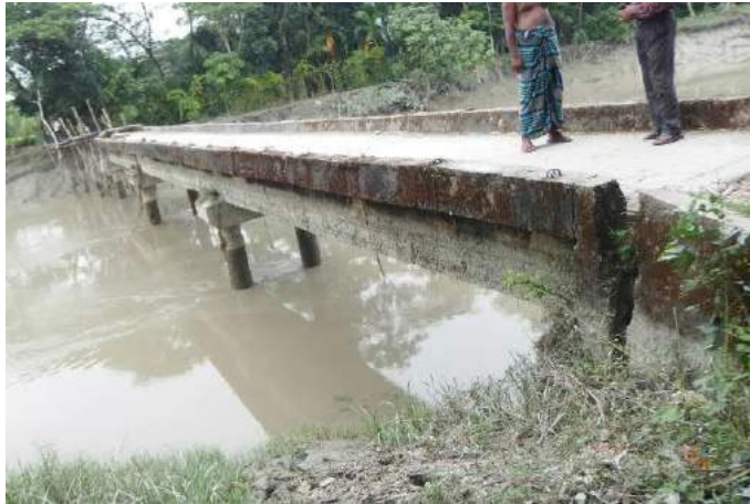
(a) General view of the Burma Bridge over Chaprashashi canal
