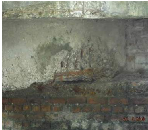
(b) Deteriorated concrete girder and rebar corrosion at abutment
