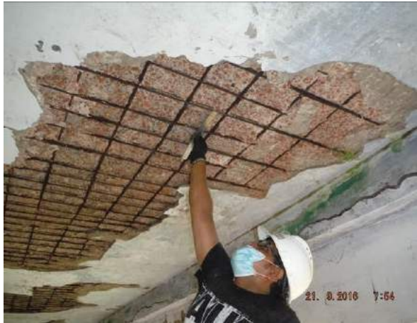
(c) Measurement of rebar spacing in roof slab concrete
