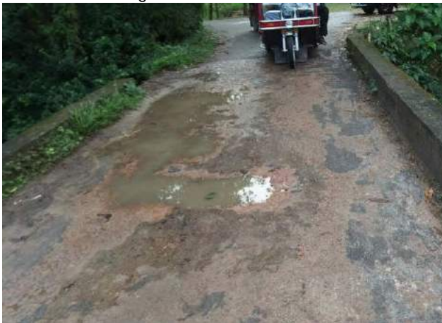
(c) Top surface of bridge deck showing abrasion of wearing course
