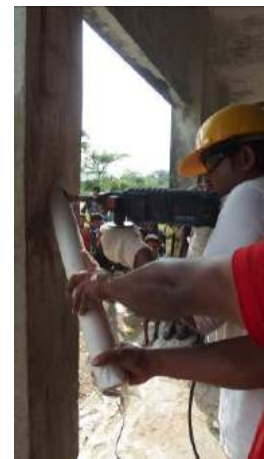
(b) Concrete dust collection from the columns in the corridor
