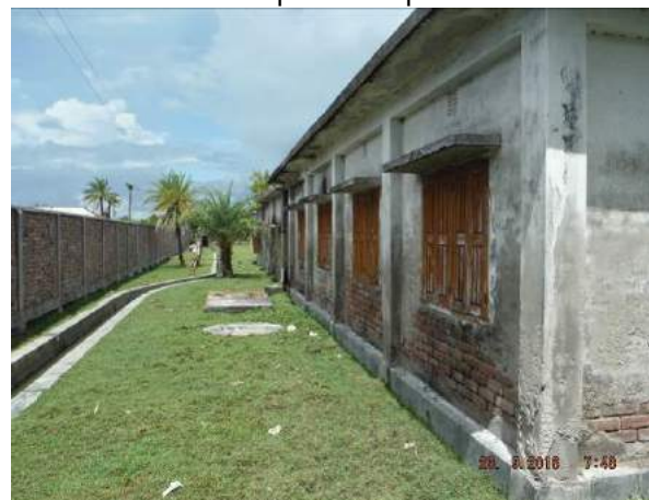
(d) Salt damage on external faces of concrete columns and masonry walls
