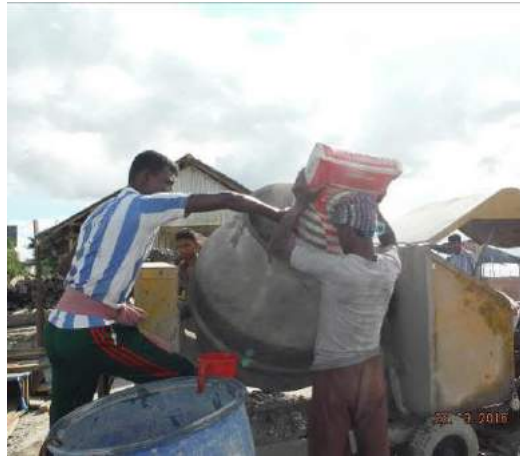
(b) Concrete 10/7 mixer - manual addition of materials
