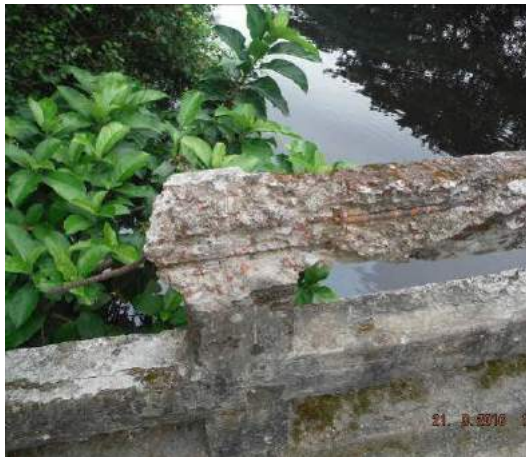
(c) Deterioration of concrete and rebar corrosion on railings
