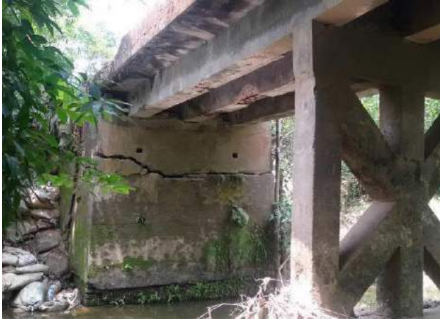
(a) Horinmara bridge – showing displacement cracking in abutments and corrosion of rebar in girders
