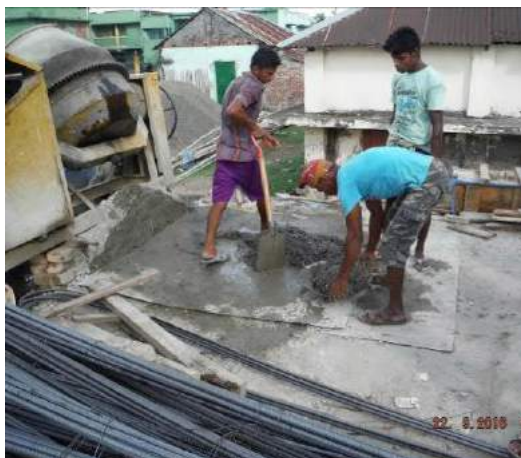
(c) Manual transportation of concrete to building site
