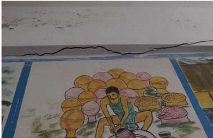
(c) Cracking and, delamination of concrete in roof slab beam
