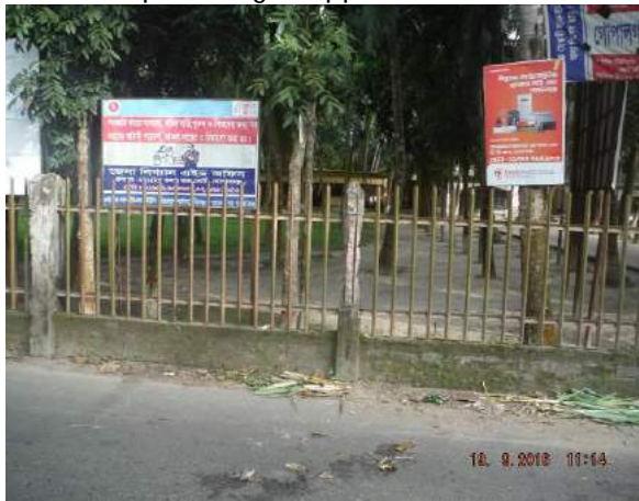
(a) Concrete column in Upazilla office fence
