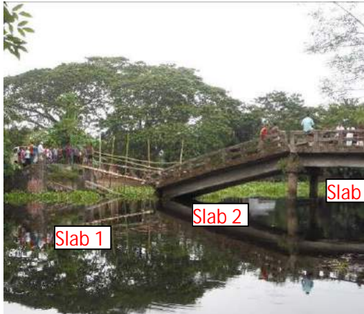
(a) Silna river Road bridge – Collapsed
