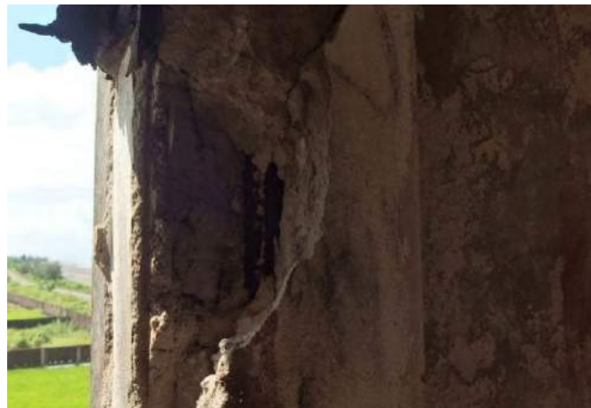
(d) Spalling of concrete and exposed reinforcement in 2 nd floor
