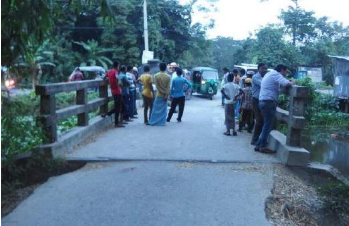
(a) General view of the box-culvert
