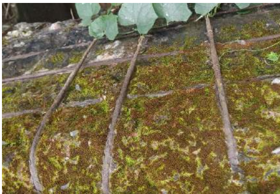
(c) Exposed rebar in outer face of south-west railing wall of the culvert
