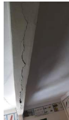
(b) Longitudinal cracking in roof slab beam
