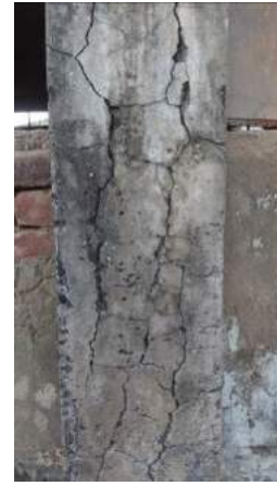
(b) Delamination and pattern cracking of concrete in column
