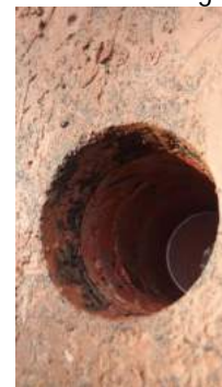
(d) Voiding at interface between wearing coarse and deck slab concrete
