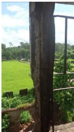
(a) Deteriorated concrete column
