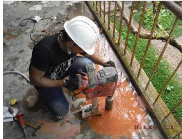
(d) Concrete core extraction from first floor base slab
