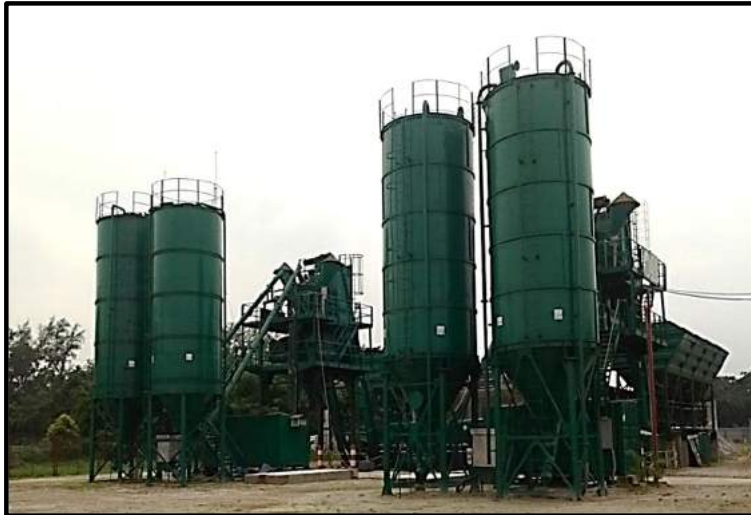
Figure 1-1 Concrete plants at the Elevated Expressway Project
