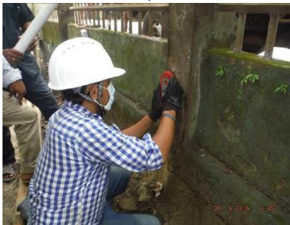
(c) NDT investigation of concrete columns
