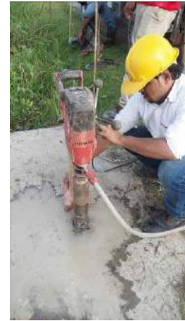
(b) Core extraction from deck slab -north end
