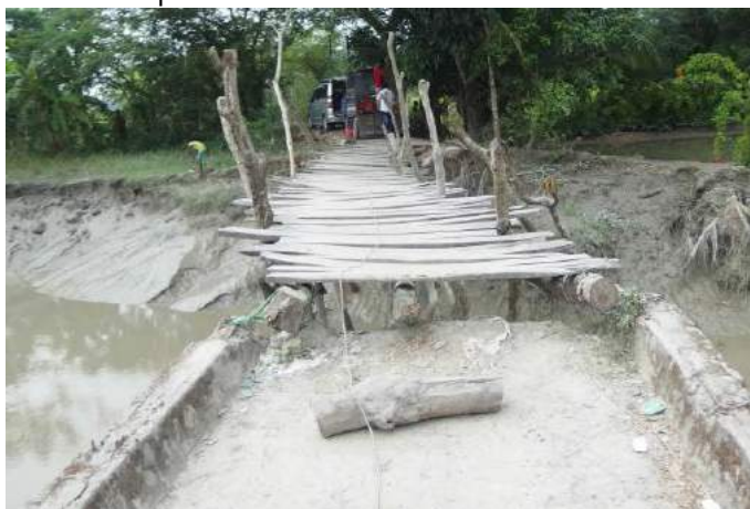
(c) Collapsed section of the bridge connected by bamboo scaffolding
