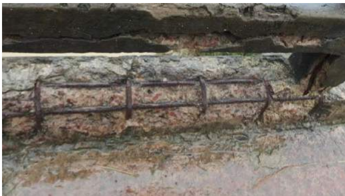
(c) Spalling of concrete, reinforcement corrosion in railings
