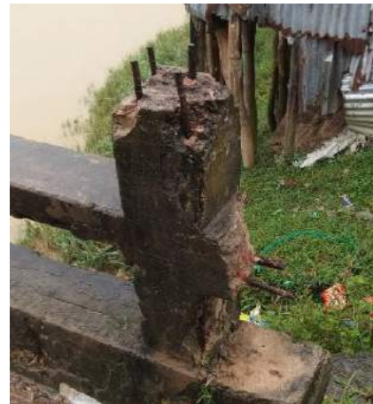
(b) Broken railings and exposed reinforcement
