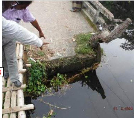
(b) Concrete spalling and reinforcement corrosion in railings
