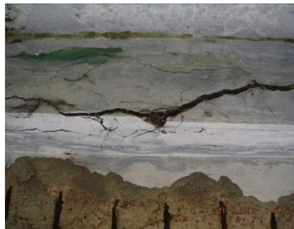
(b) Location of concrete dust samples on pier-1
