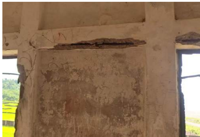
(b) Concrete spalling and rebar corrosion in lintel beams
