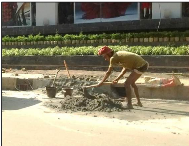
Figure 1-2 Hand-mixed concrete at local drainage works in Dhaka city
