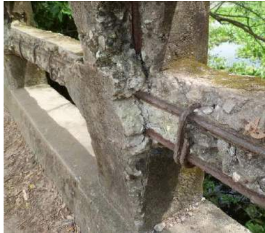
(b) Concrete spalling, delamination and reinforcement corrosion in railings
