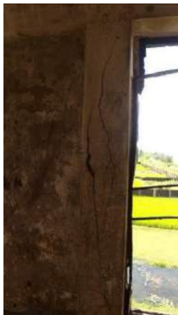
(c) Cracking and, delamination of concrete in 1 st floor columns
