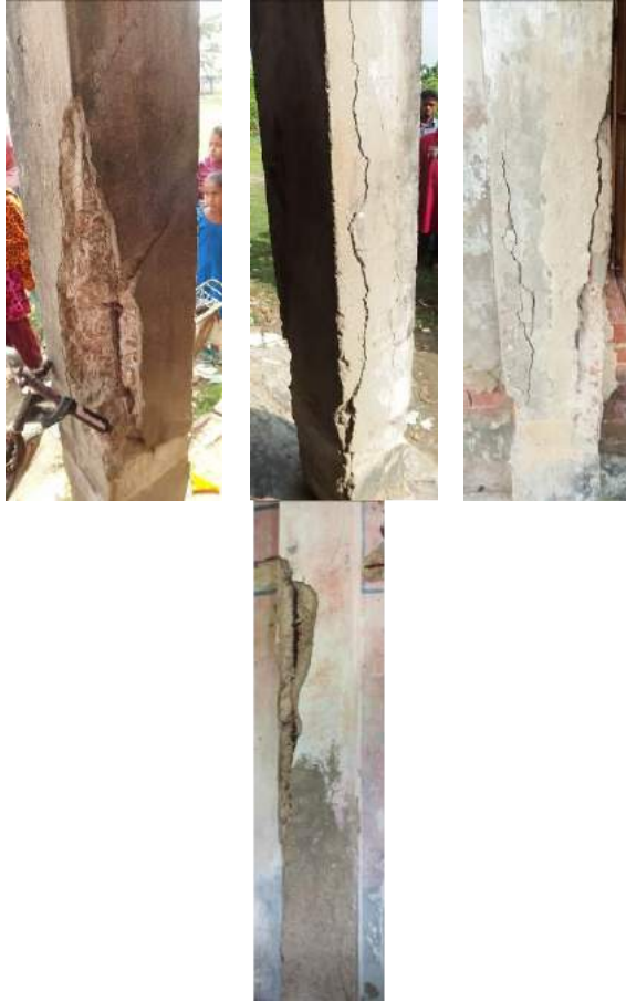
(c) Extensive corrosion induced damage of various columns in the school building
