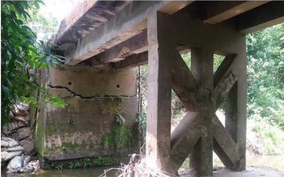
Horinmara Bridge – Shear failure of Abutments
