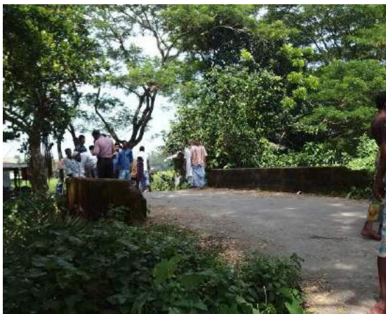
(a) General view of the box-culvert
