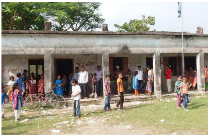
(a) General view of the Primary School building
