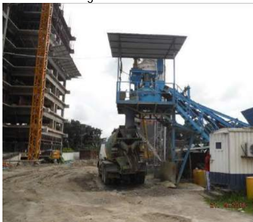
(c) Concrete batching plant at site
