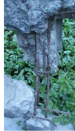
(b) Severe damage to rail post
