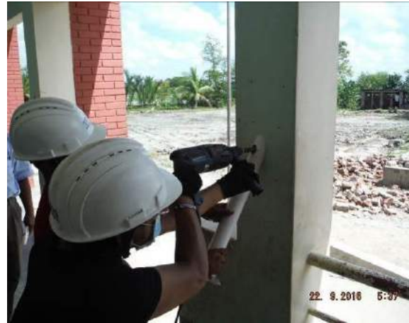
(b) Collection of concrete dust samples in column
