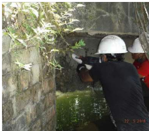
(d) Collection of concrete dust sample on side face of girder
