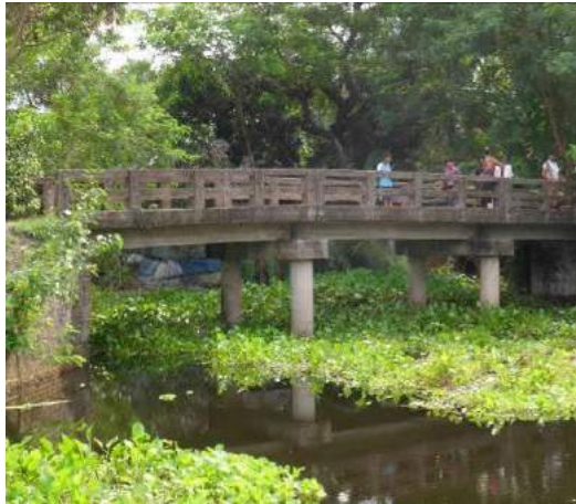
(a) Road bridge – 20m length
