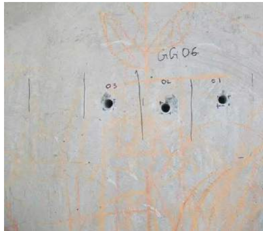
(b) Location of concrete dust samples on pier-1
