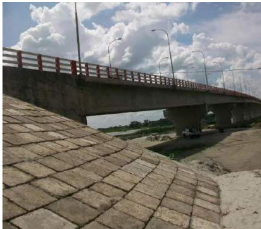
(a) Chapail road bridge on Modhumati river
