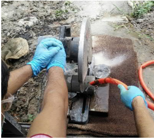
(a) Concrete saw cutting
