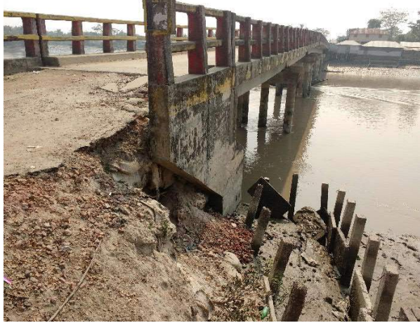
Photo: Site 21, Structure Inspection
