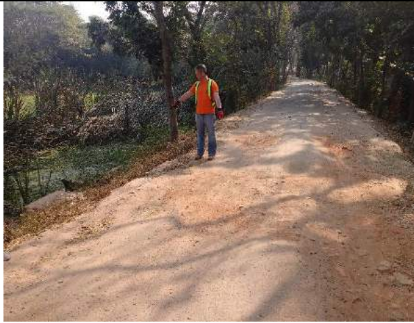
Photo: Site 15, Structure inspection
