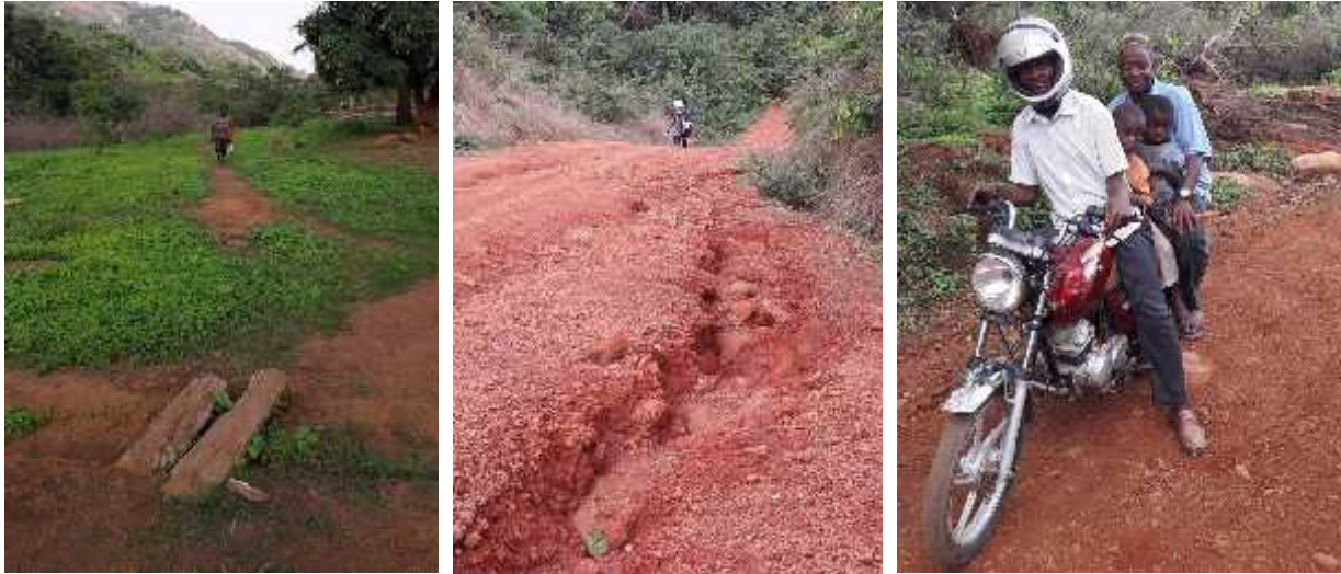
Figure 13 (left): Start of the footpath near Kamba which is considered for upgrading.
