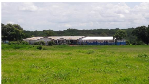
Figure 13 (left): The school-building in Batkanu.
