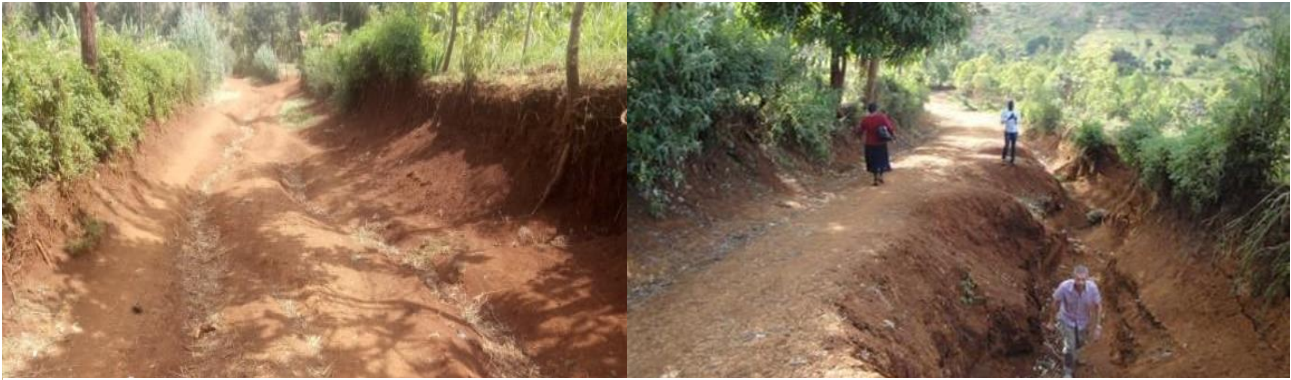
Figure 1: Steep roads with no drainage in Meru, Kenya
