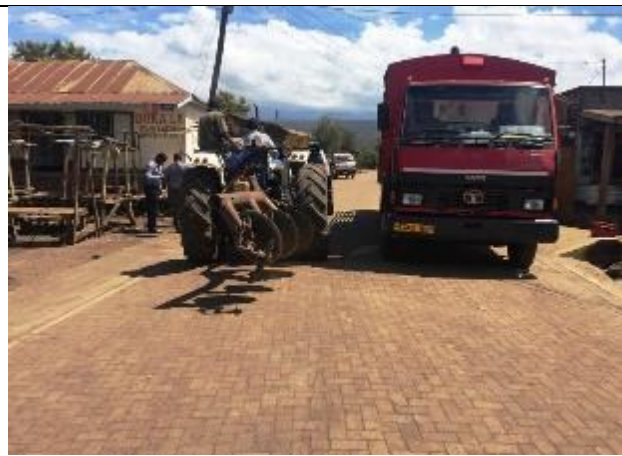
Good performing block paving section, and typical traffic
