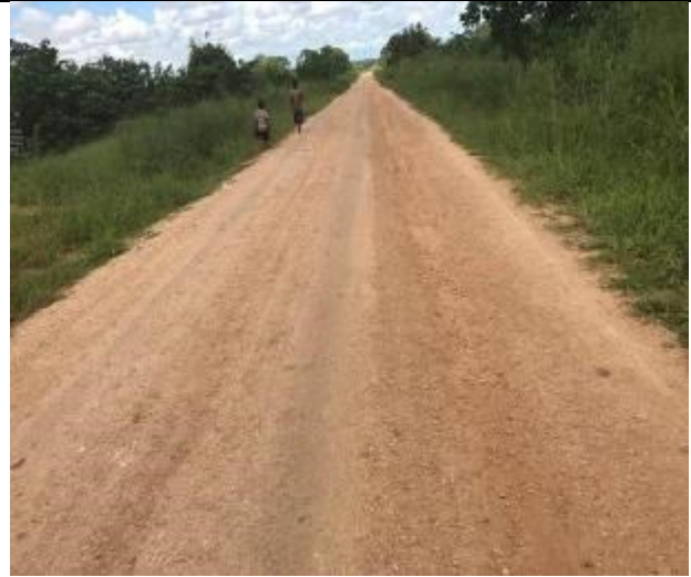
Gravel wearing course sections: Severe rutting in wheel paths
