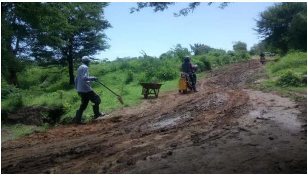
Figure 14 Slippery muddy/boggy spot on Access Road 4, Kauthilini
