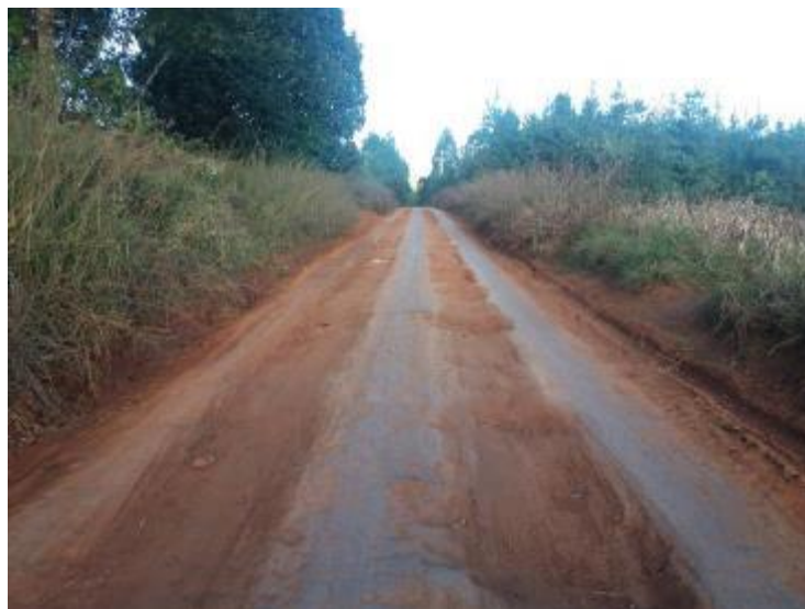
Figure 17 Slippery, rutted and boggy spot on major route to Madeke, A1
