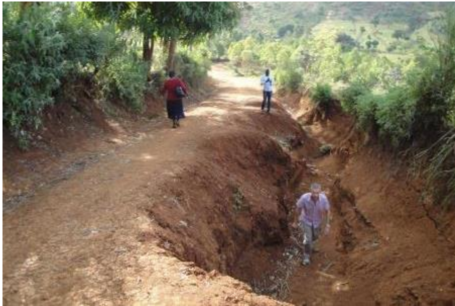
Figure 12 Extreme gully and road with narrowing on Access Road 4, Miathene
