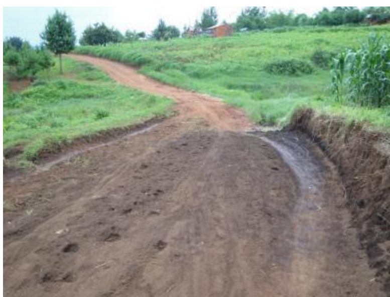
Figure 15 Soft/Boggy spot leading to water crossing in Matola
