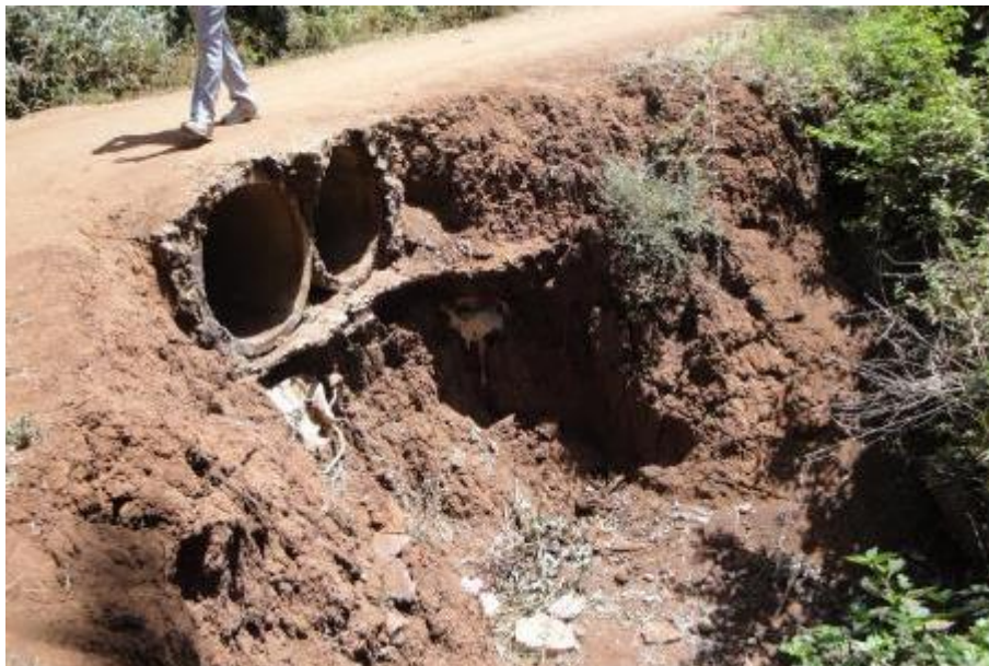
Figure 12 Extreme gully and road with narrowing on Access Road 4, Miathene
