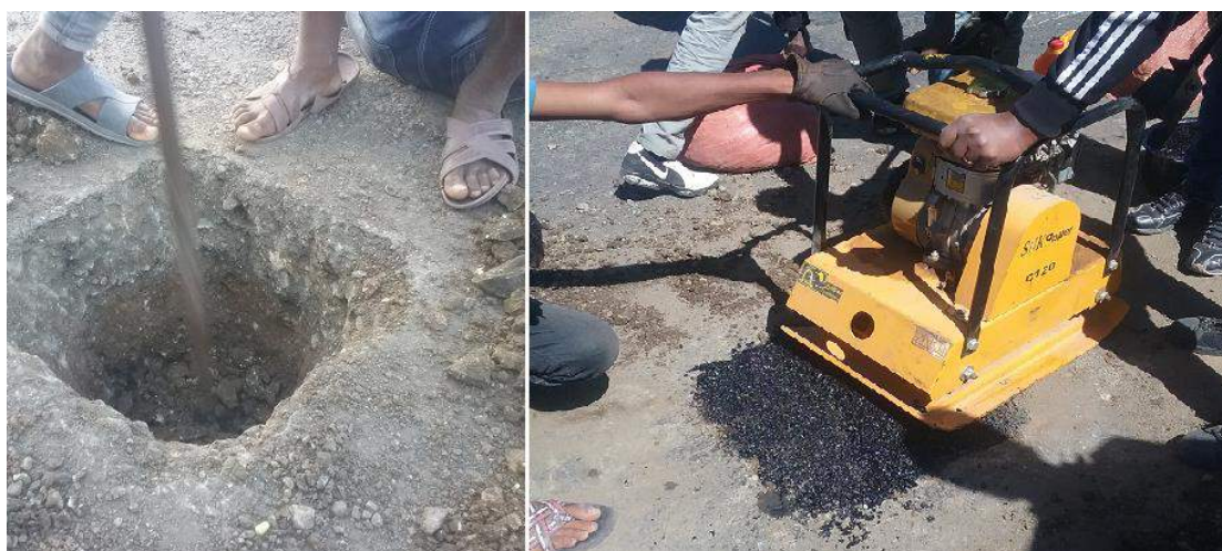
Figure 2-4: Test Pit trench for sampling and compaction for reinstatement
