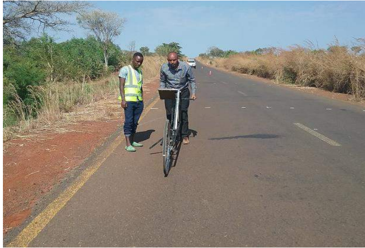
Figure 4-3: Roughness measurement using MERLIN for Assossa - Kumruk trial section
