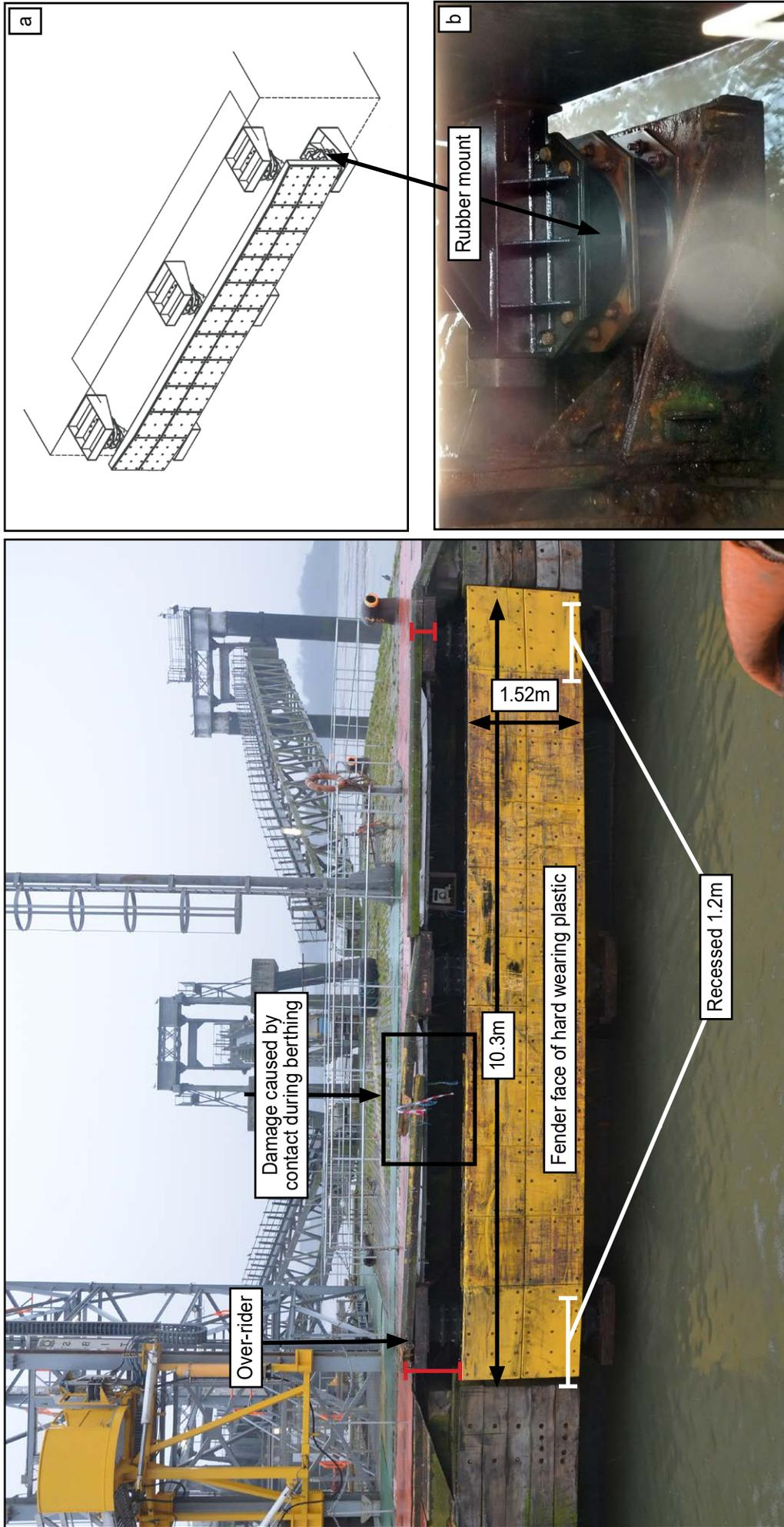
**Figure 9:** North oil stage fender (**inset a:** Isometric view and **inset b:** Rubber mount)
