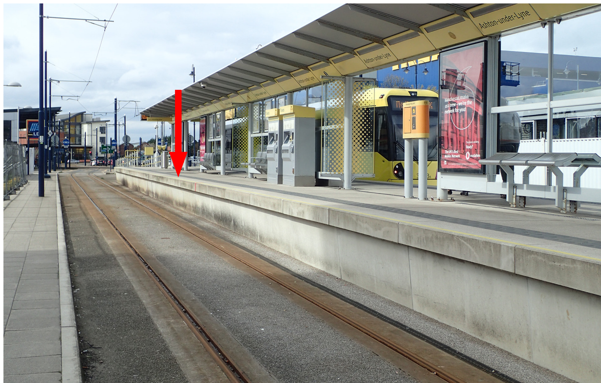
Figure 3: Platform B at Ashton. The red arrow indicates the point at which the passenger was standing when he fell from the platform.
