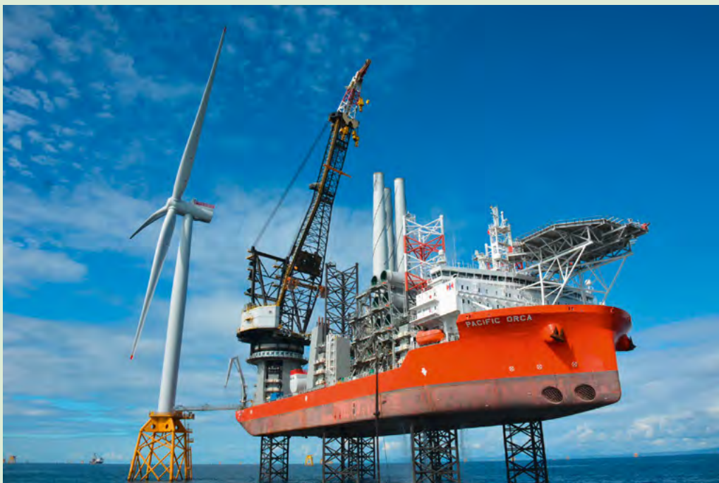
Pacific Orca installation vessel (Image: JBray)
