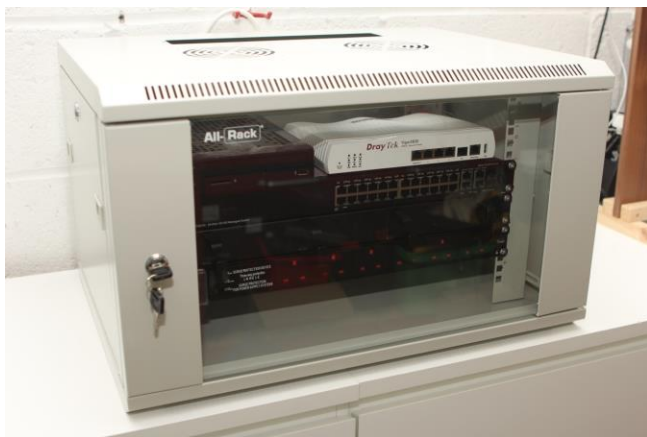
Figure 7 - Example of a cabinet housing the LAN Server, Network switch, LAN router and the security sticker placement
