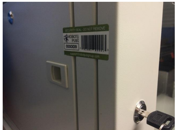
Figure 7 - Example of a cabinet housing the LAN Server, Network switch, LAN router and the security sticker placement
