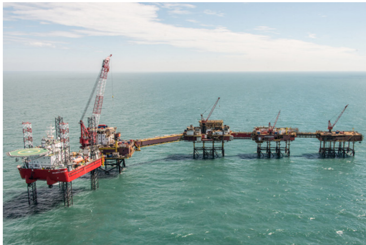
Seajacks Leviathan jack-up accommodation work vessel at Viking Bravo completing the transition to cold suspension in 2017
