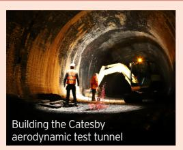
Adapted from a 1.7 mile straight and flat former railway tunnel, the Catesby Tunnel will allow full scale vehicle testing in constant conditions due to the naturally stabilized environment generated from being underground. The tunnel will also be fitted with automated turntables at either end to allow for return testing. The Catesby Aero Research Facility will also lead to the creation of a 4.5 acre science park with offices, workshops
