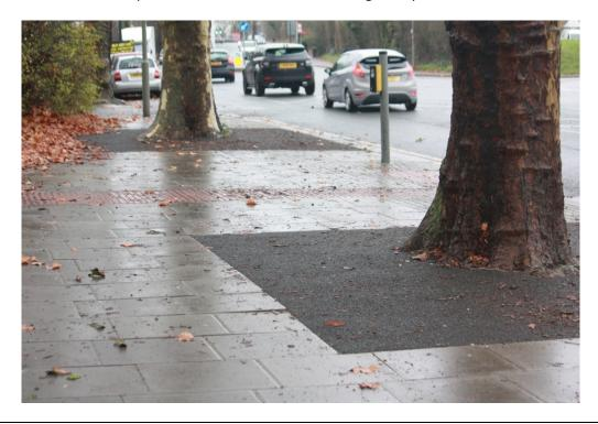
ii. Flexible pit size with rubber crumb insert narrow pavement.
