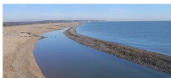
Pevensey Bay flood defences, Sussex 3,100 homes protected
