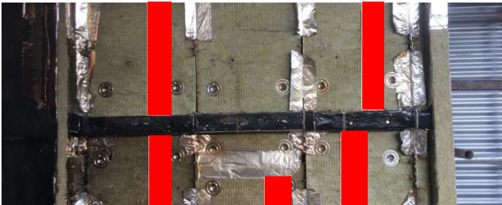
Figure 12 – 3 rd cavity barrier from return wall following removal of the rainscreen
