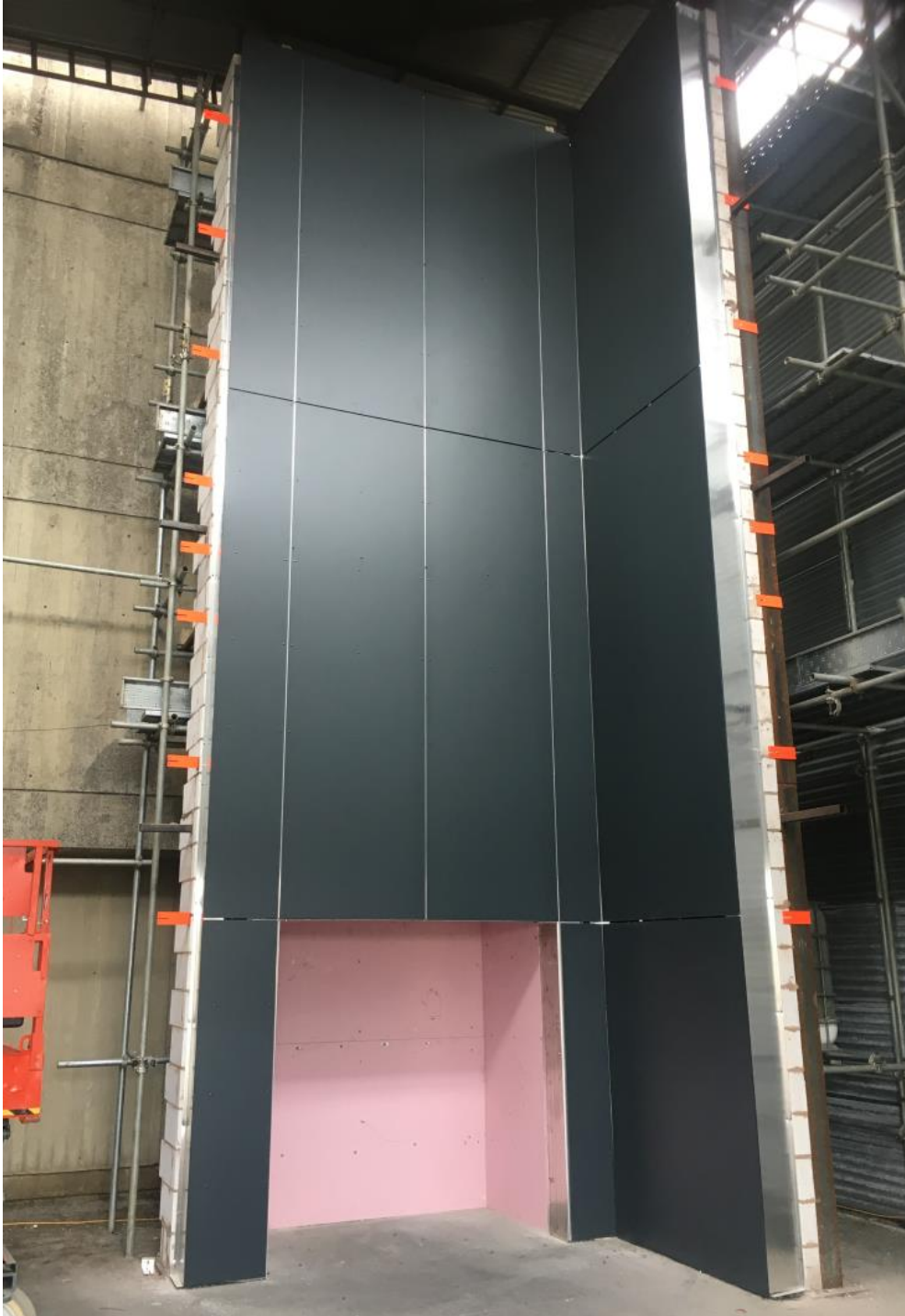
Figure 2 – Finished installation on the test wall
