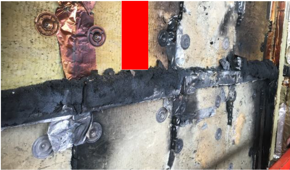
Figure 11 – 3 rd cavity barrier from main wall following removal of the rainscreen
