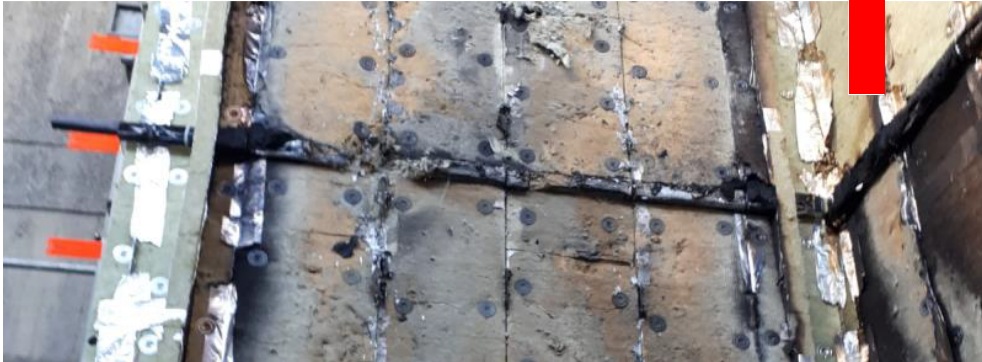
Figure 9 – 2 nd cavity barrier from main wall following removal of the rainscreen
