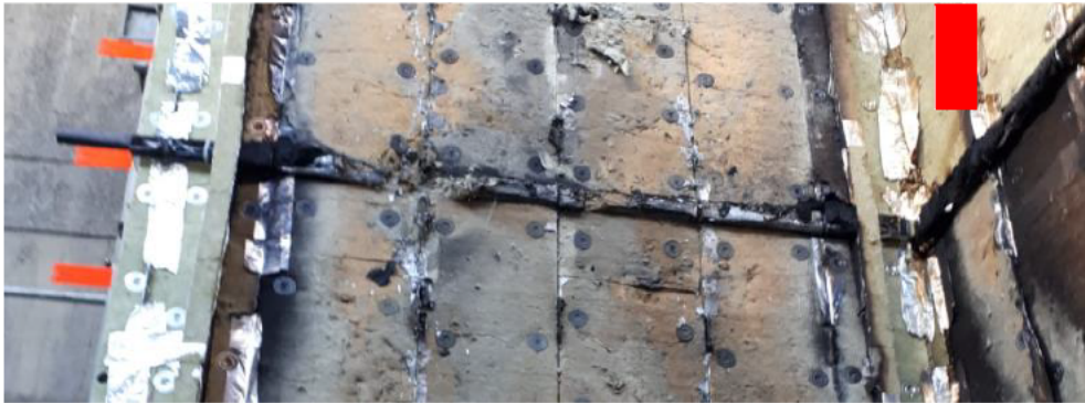
Figure 26 – 2 nd cavity barrier from main wall following removal of the rainscreen
