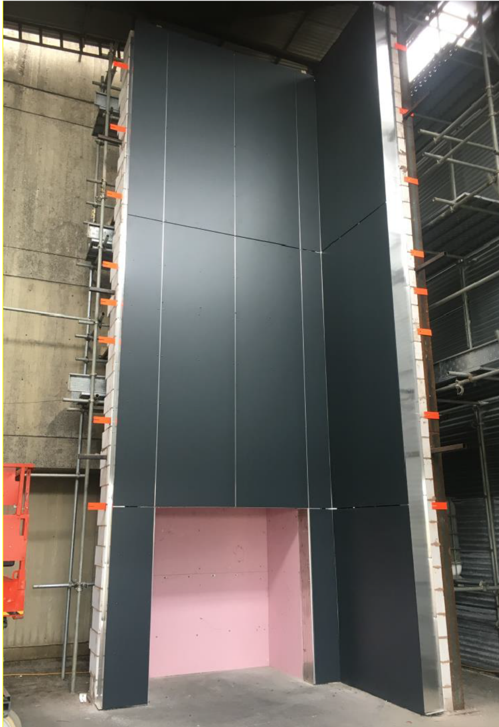
Figure 2 – Finished installation of cladding system under test
