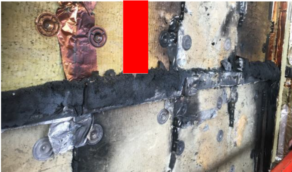
Figure 28 – 3 rd cavity barrier from main wall following removal of the rainscreen
