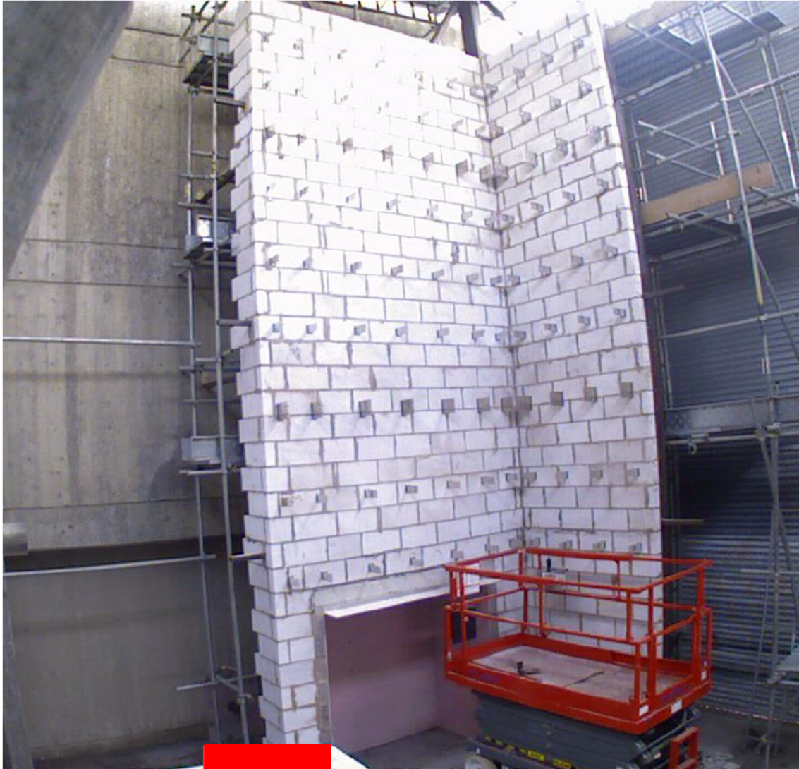
Figure 17 – Masonry wall with helping hand brackets installed
