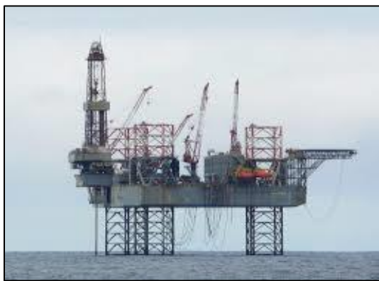
Figure 2.14 – Ensco 100 Drilling Rig
