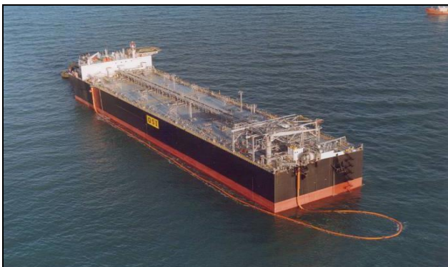
Photo 4 - Oil Storage Installation
