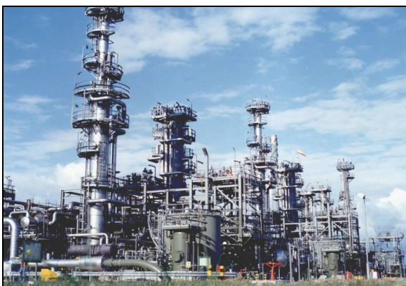
Photo 5 - POA Gas Terminal
