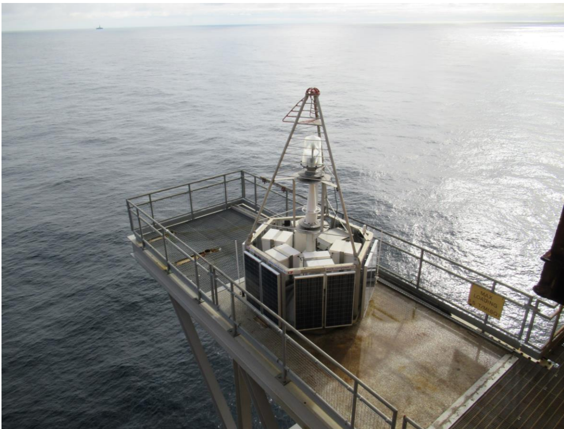
Ninian Northern Navigation Aid installed to mark the platform's location during the idle phase
