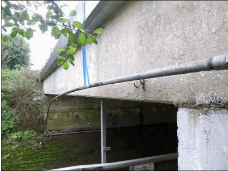
009. North Fascia & Parapet Beam
