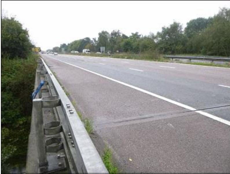
011. View of Carriageway Looking East
