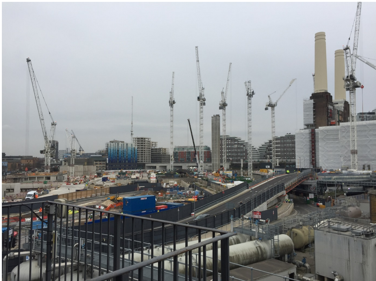
Figure 2: Battersea Power Station development, boundary with Northern Line extension.
