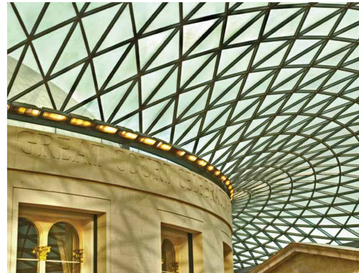
Glass roof of the Great Court at the British Museum with the Reading Room building in the foreground, London
