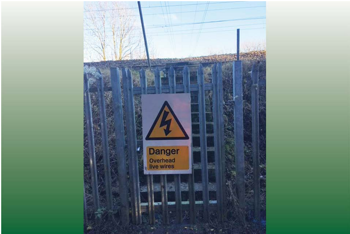
The access point used by the track workers (image courtesy of Network Rail)
