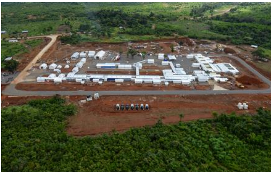
Figure 4: The Kerry Town Treatment Centre in Sierra Leone near the capital Freetown.
