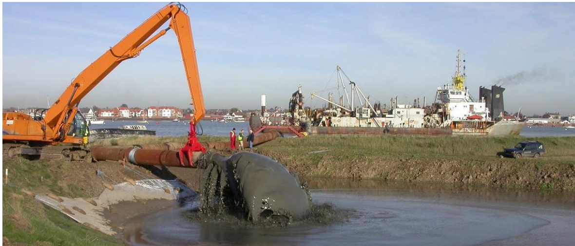
Figure 5: Large-scale (550,000m 3 ) beneficial use of dredged silt for pre-breach land-forming at Allfleet's Marsh on Wallasea Island.
