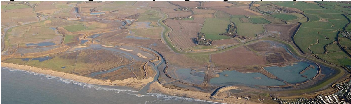
Figure 3: Aerial image of Medmerry managed realignment (January 2014).
