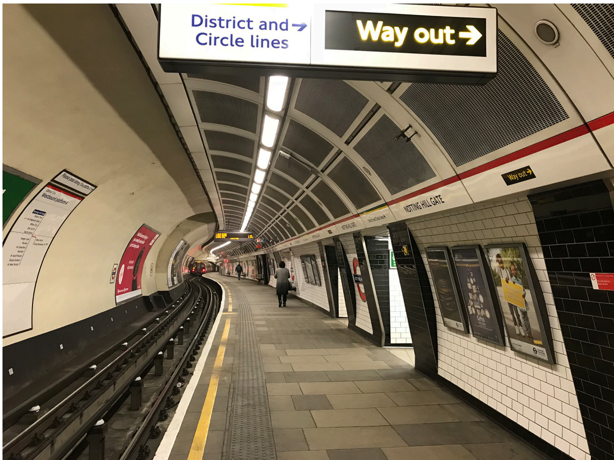
Figure 2: View from the east (tailwall or rear) end of platform 4 at Notting Hill Gate facing west, showing the reverse curve
