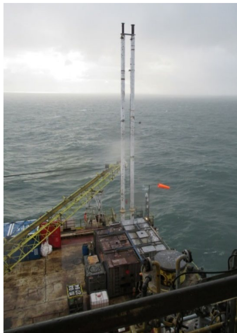
Figure 2.2 – Photograph of Vent Stack, SW corner of Platform
