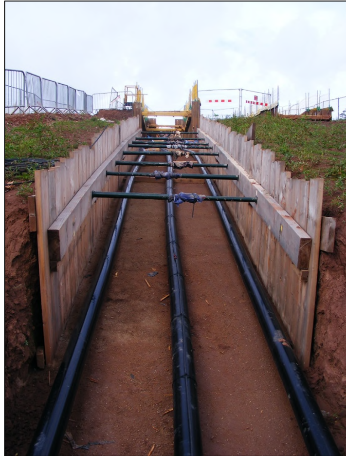
Installation of ducts ready for cabling
