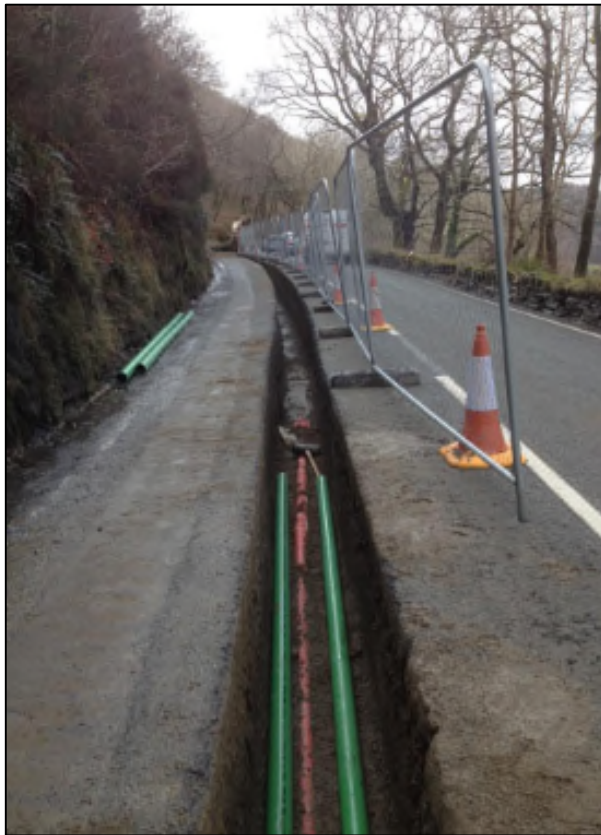
Works within single carriageways – traffic controlled
