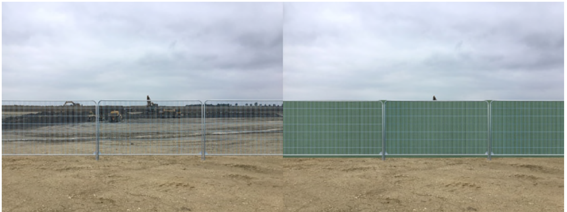
Figure 3: Illustrative example of borrow pit security fencing without mitigation (left) and with mitigation (right)
