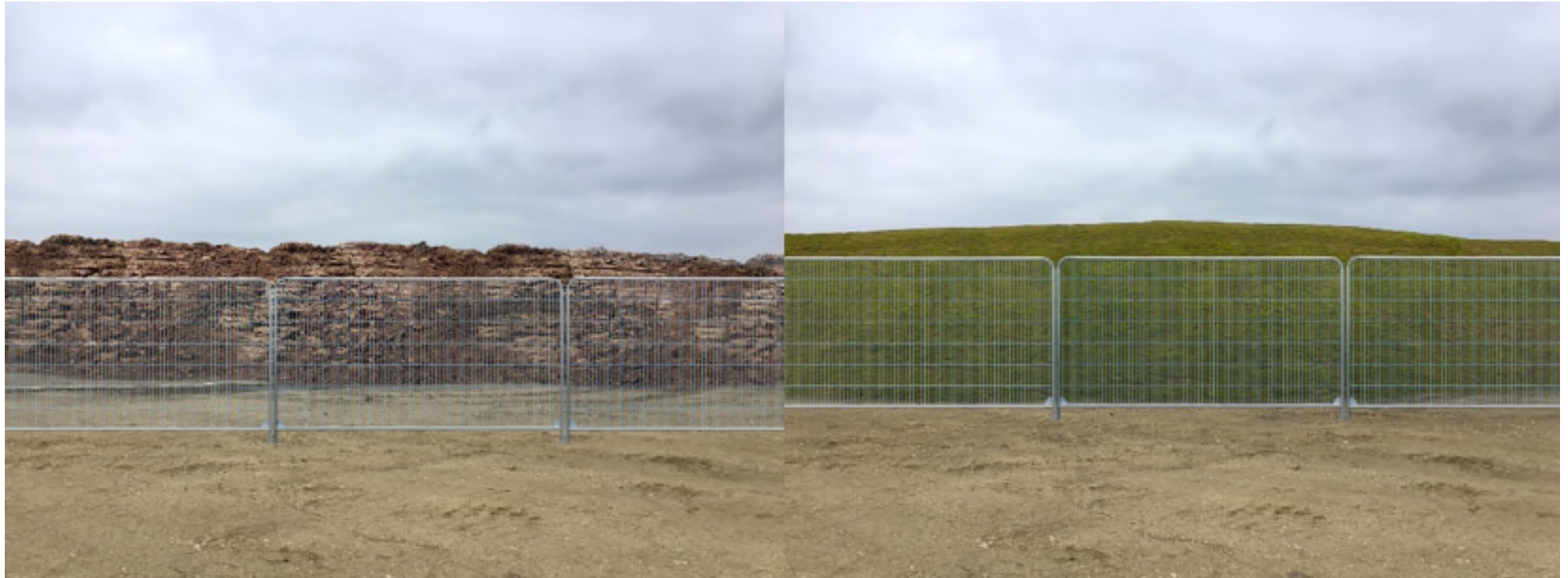
Figure 4: Illustrative example of typical borrow pit boundary soil stockpiling (seeded in the right hand image)
