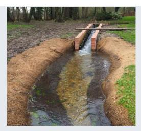
Larinier fish pass installed at Holbury with eel substrate attached to right side of the fish pass
