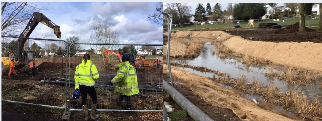
Flows returning to a newly meandered channel and new channel with re-profiled banks
