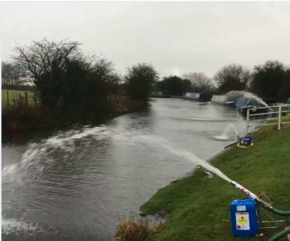
Officers deploying hydrogen peroxide to a section of deoxygenated canal.
